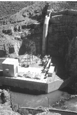
Buffalo Bill Powerplant in the canyon downstream from the dam
