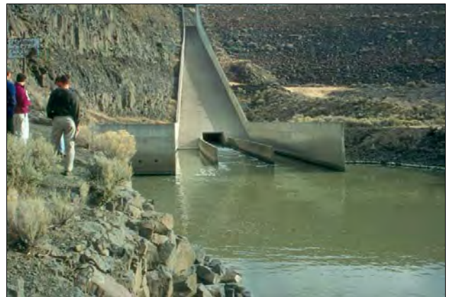
Photo 3-1. Bowman Dam spillway.
