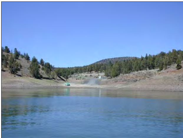
Photo 3-14. County Boat Ramp.
