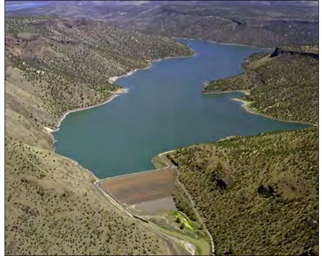
Photo 1-2. A view of Bowman Dam and Big Bend Campground in the foreground and Prineville Reservoir eastward.
