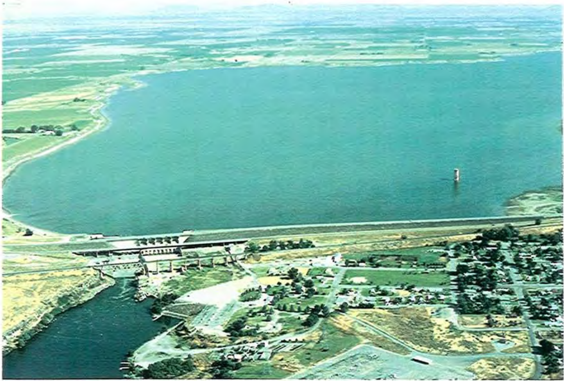
American Falls Dam
