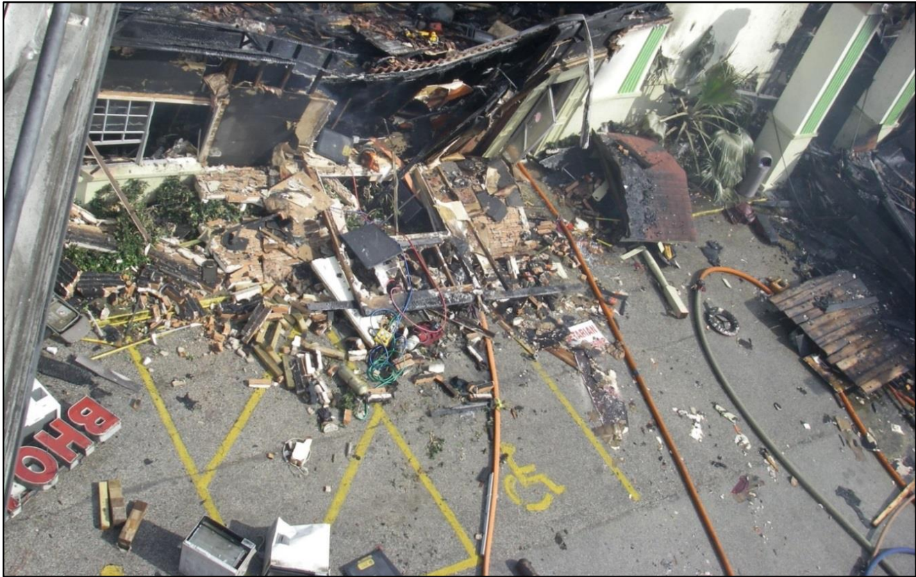
Photo 7. The front façade collapsed at 1303 hours striking fire fighters and officers assigned to the Rescue Group. These members were quickly removed by other fire fighters who picked up the façade and pulled the trapped fire fighters and officers out. (Photo courtesy of the fire department)
