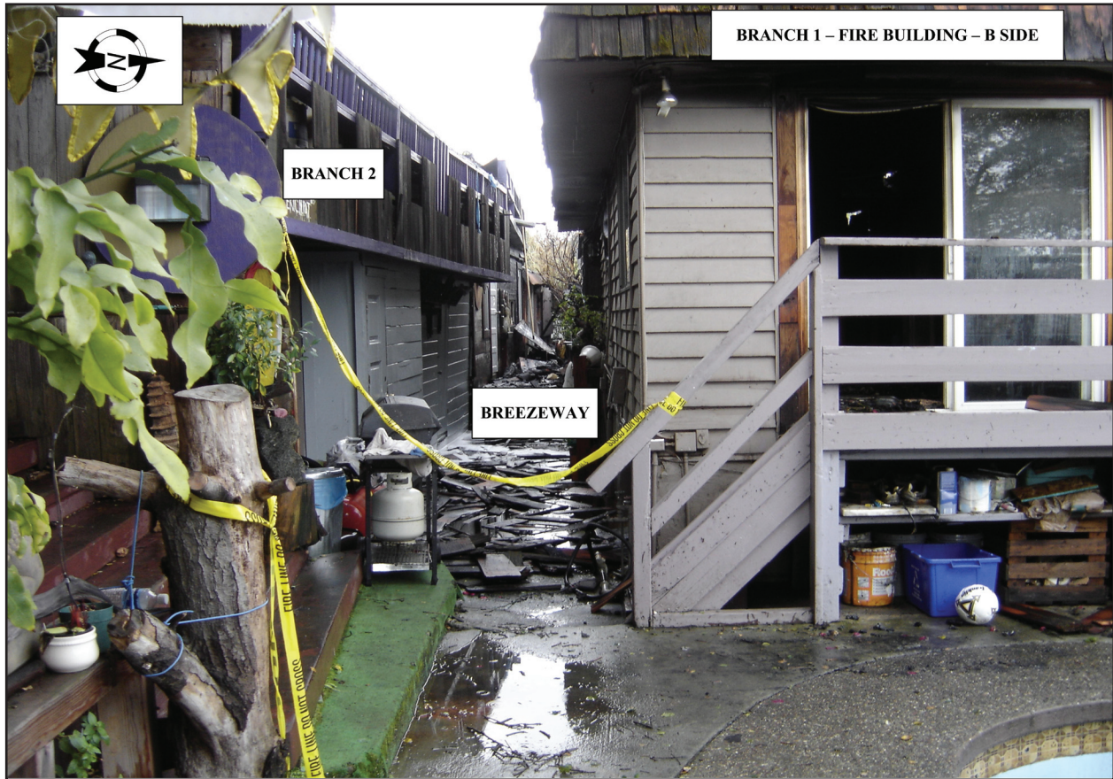
Photo 1. Photo showing Branch 1 and Branch 2 Photo courtesy of the fire department
