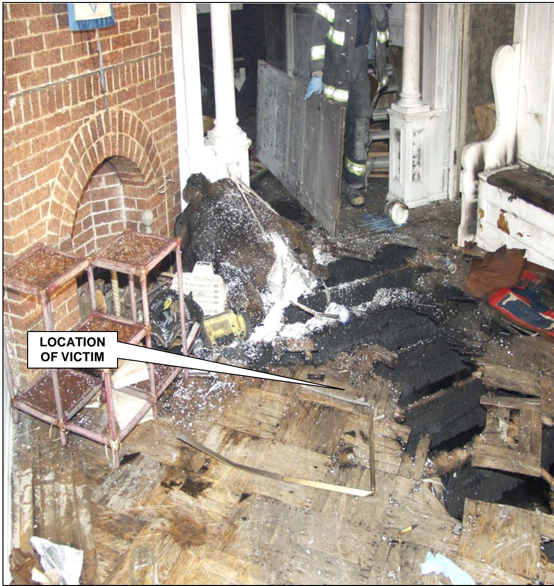
Photo 4. Living room floor
