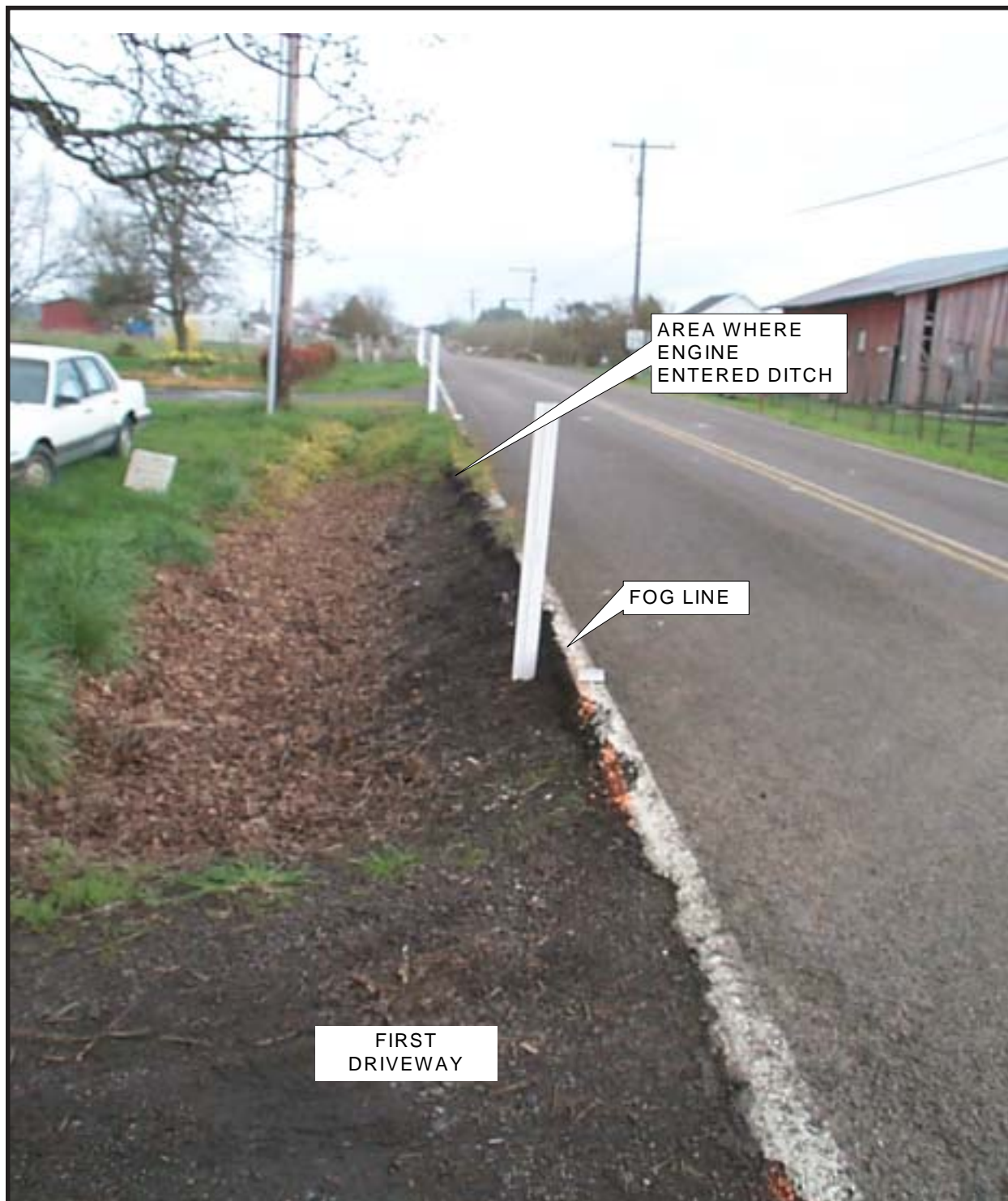
Photo 2. Ditch 40 inches deep
