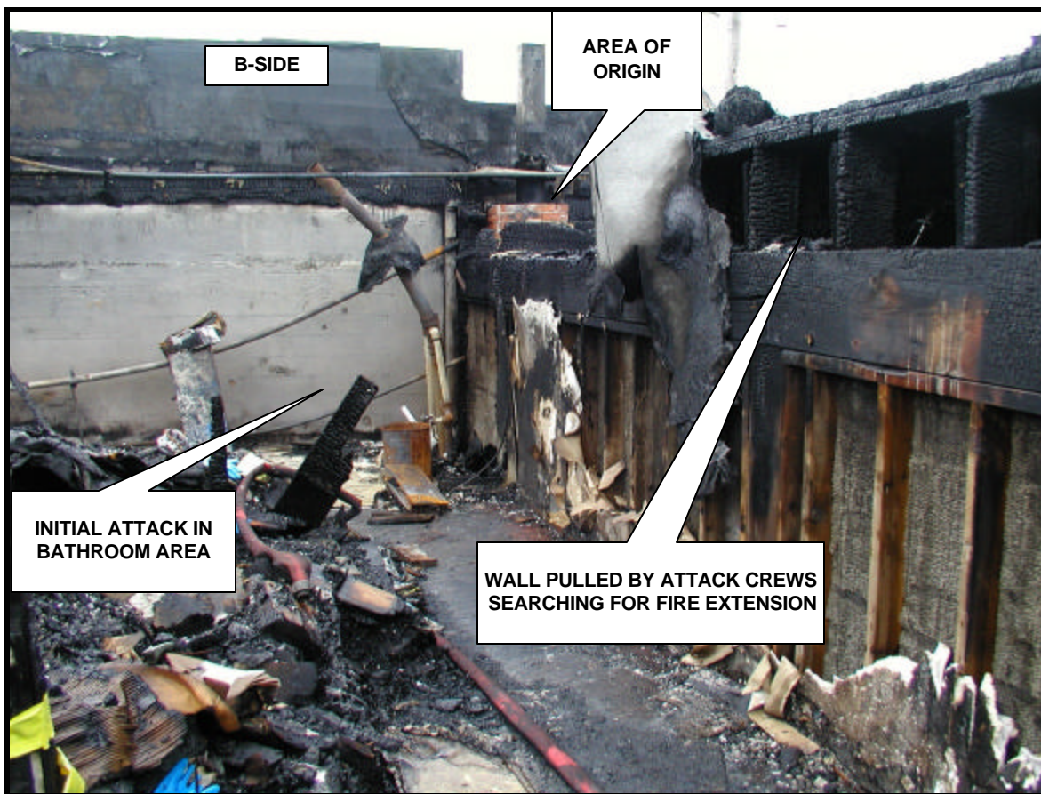
Photo 1. North-East corner of mezzanine where attack crews were operating
