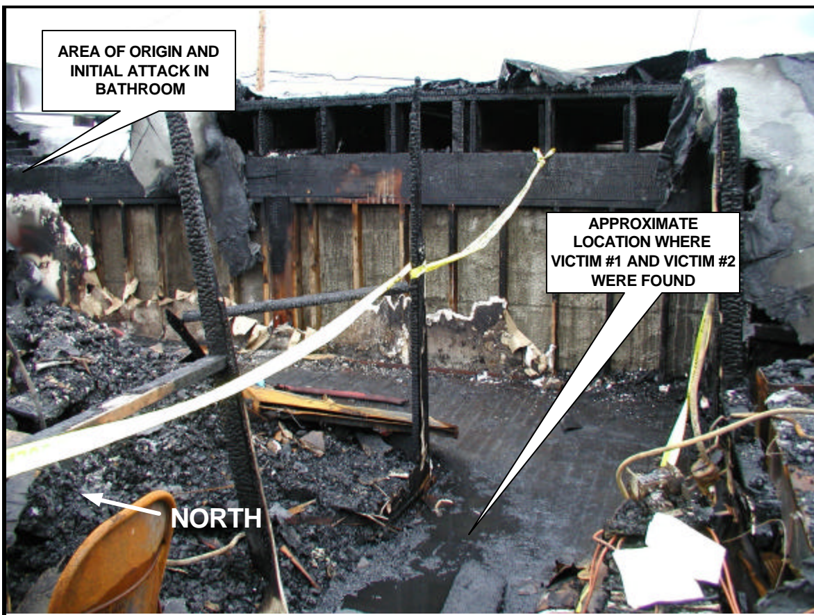
Photo 2. View of east wall on mezzanine
