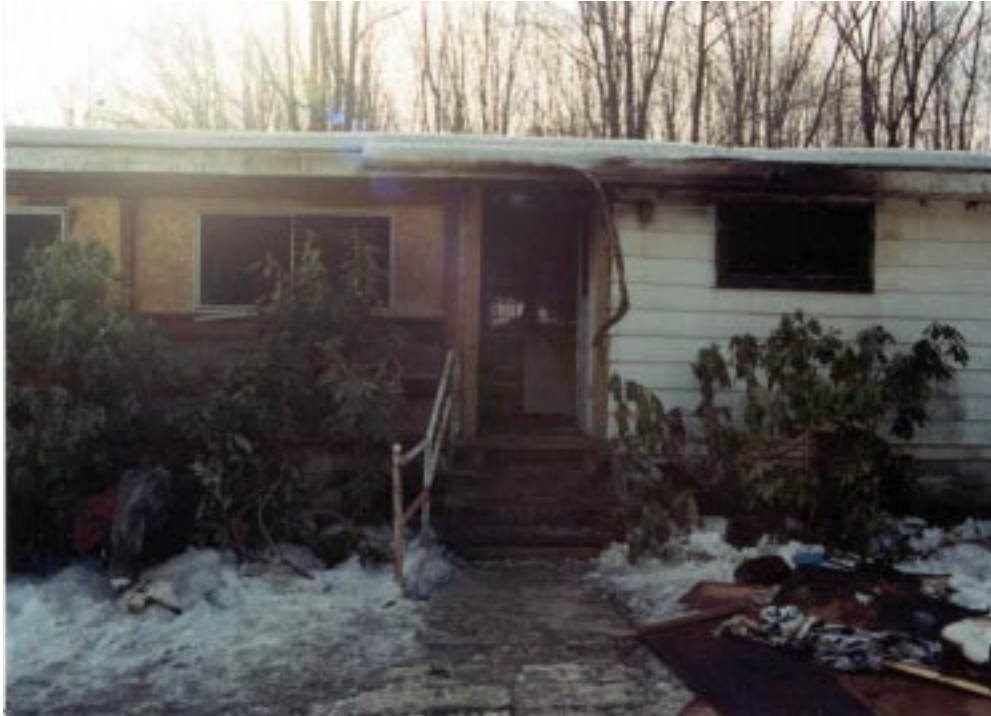
Photo 1. Front Door Entrance to Mobile Home (Side 1)
