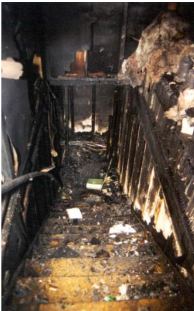
Photo 7. Stairway Connecting Addition to Basement
