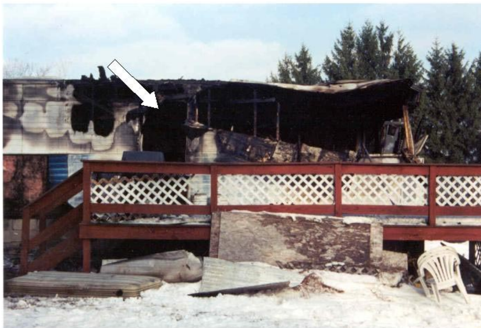
Photo 4. Doorway Into Corner Bedroom (Side 3)
