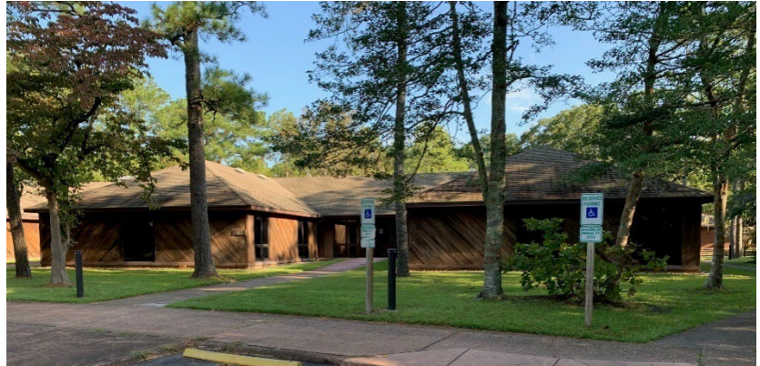
Figure 22. Reserve Northern Office
