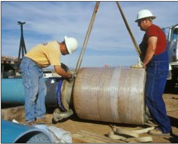
Figure E2a: Assembling the wedge-wire fish screen system.
