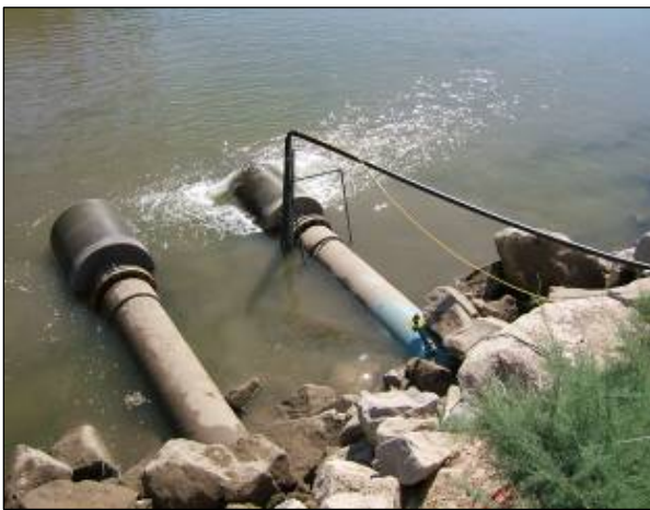
Figure E2b: In situ hydraulic testing of the wedge-wire screens.
