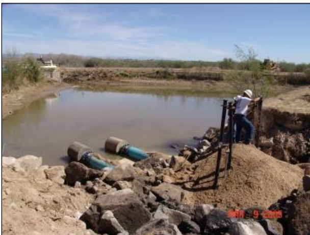
Figure E2c: Installation of the wedge-wire fish screen system.
