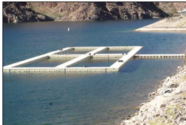
Figure C9b: Assembled docking place alongside hatchery.
