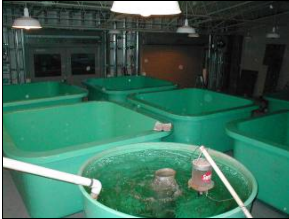
Figure B6: New tanks installed in Lake Mead SFH native fish room.
