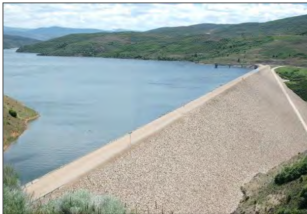
Photo 1-4: Jordanelle Dam looking East
