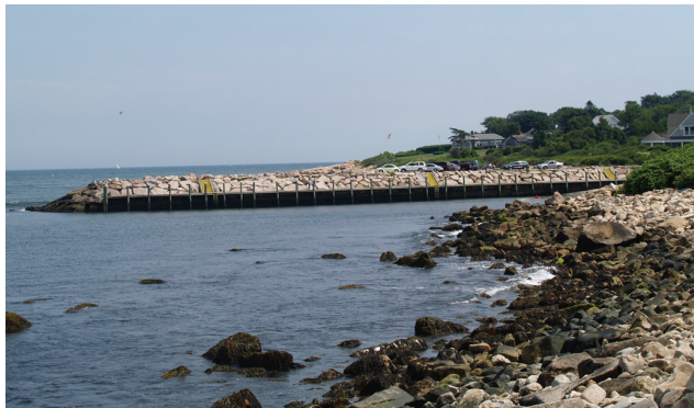
Figure 8.16. This bulkhead at State Pier #5 in Narragansett provides a sheltered cove to tie up, launch a boat, fish, or scuba dive. Human-made structures are designed to prevent erosion and provide sheltered areas for human use. Photo by Malia Schwartz.
