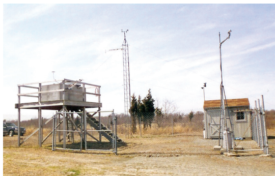
Figure 4.2. The NBNERR weather station on Prudence Island. Photo from NBNERR photo library.
