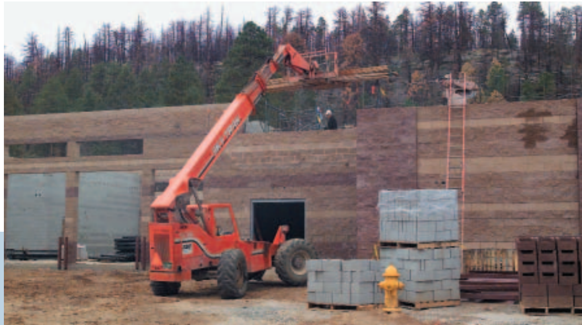
Appropriate construction equipment selection reduces site environmental impacts.
