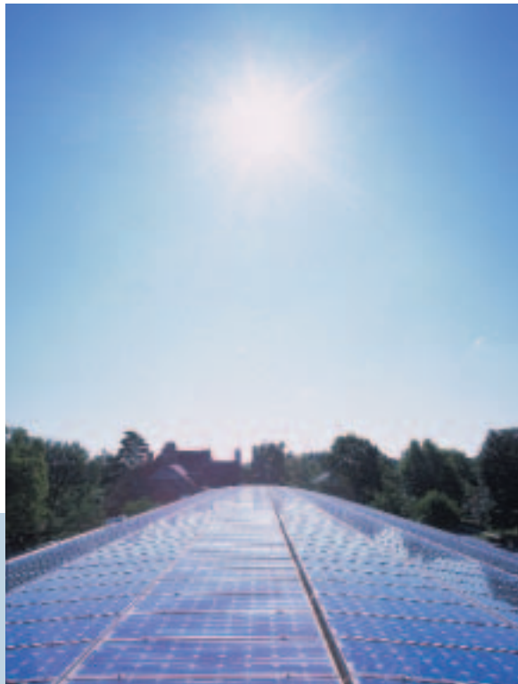
60-kW roof-mounted PV system offsets 50% of the annual electrical load of the Lewis Center for Environmental Studies at Oberlin College in Oberlin, Ohio.
