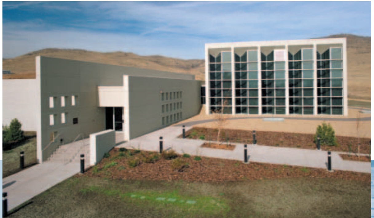
The long east/west axis, undulating Trombe wall providing passive solar heating and daylighting, and the horizontal architectural elements shading the Trombe wall in summer are sustainable building design features of the National Renewable Energy Laboratory Visitor's Center in Golden, Colorado.
