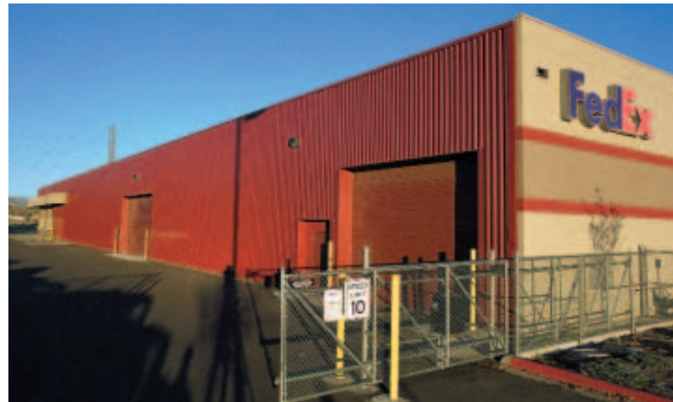
Red transpired solar collector installed as a retrofit on the entire south wall of the Federal Express building in Englewood, Colorado. Almost any dark color can be used for the perforated wall, giving some architectural flexibility. Choosing colors other than black has only a small effect on the system performance.
