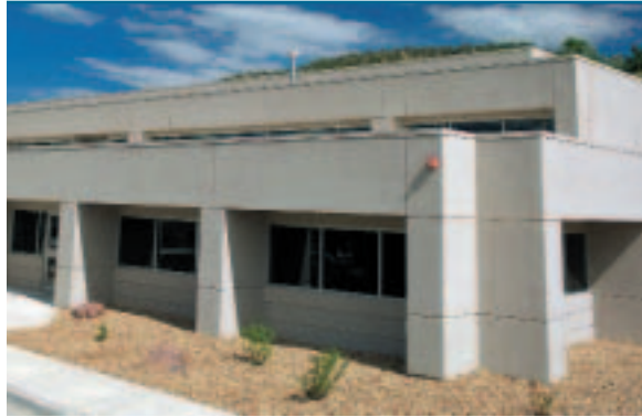
Overhangs and vertical fins on the lower windows and the overhangs on the clerestory windows provide shade to maximize daylighting and minimize summer solar gains to the Thermal Test Facility, National Renewable Energy Laboratory, Golden, Colorado.
