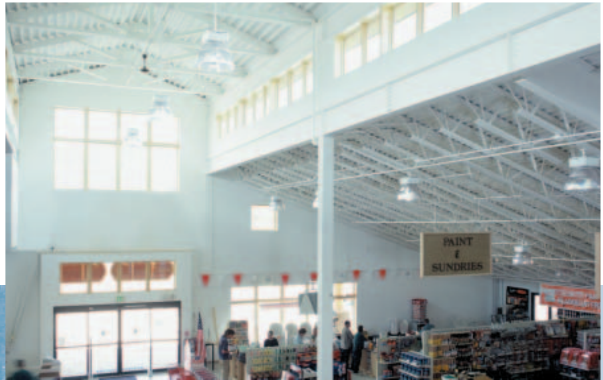
Daylight entering the space through clerestory windows is reflected off the bright white ceiling to provide diffuse daylight throughout the ACE Hardware Store at the BigHorn Center in Silverthorne, Colorado.
