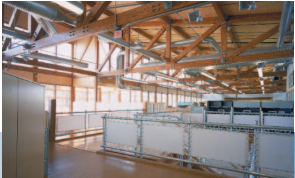
Unfinished pressed fiberboard and the lack of interior finishes and fixtures reduce resource use and indoor air pollutants in the Chesapeake Bay Foundation's Phillip Merrill Environmental Center in Annapolis, Maryland.
