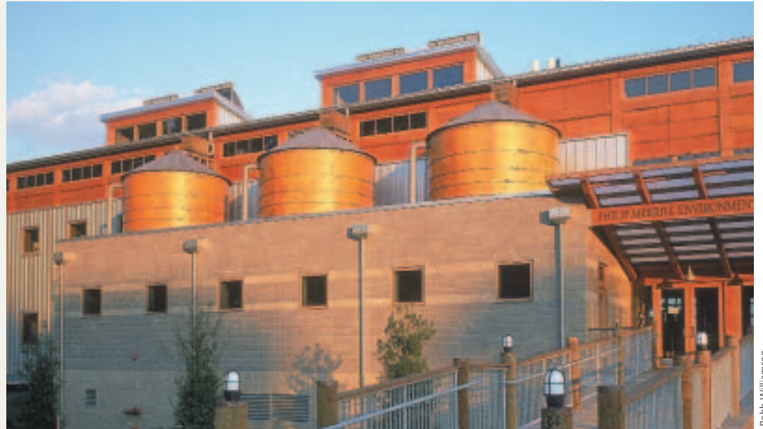
A rainwater harvesting system on the Chesapeake Bay Foundation's Philip Merrill Environmental Center in Annapolis, Maryland, captures rainwater for use in fire suppression and in the building's sinks.
