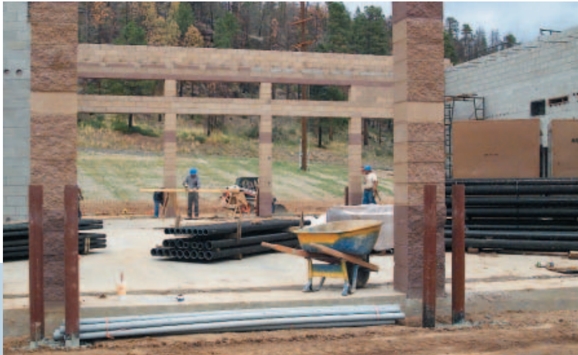
An organized, well-managed construction site promotes safety.
