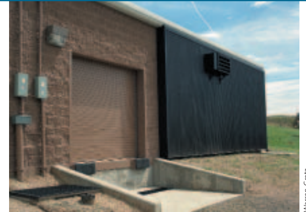
The transpired solar collector is the only heating system for this small waste handling facility at the National Renewable Energy Laboratory in Golden, Colorado.
