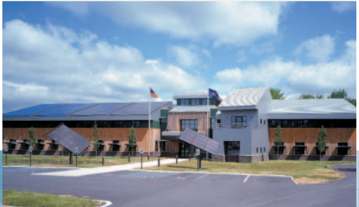
The Cambria Office Building, which houses Pennsylvania's Department of Environmental Protection, is a high-performance office building that incorporates energy efficiency and renewable energy design strategies.
