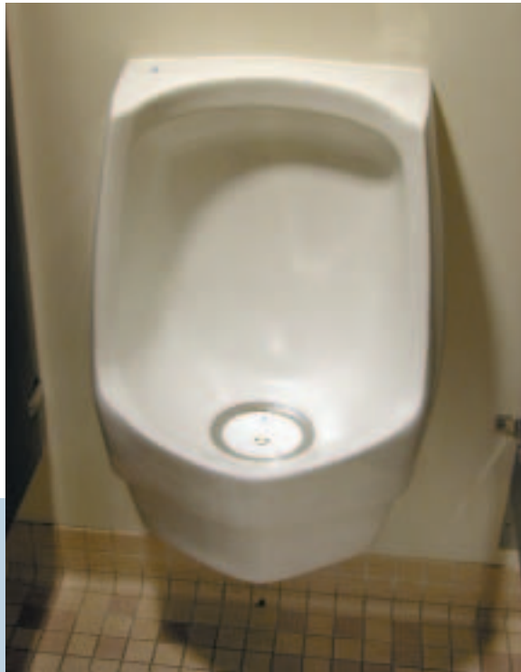
Waterless urinals represent the most water-efficient urinal option.
