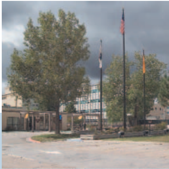
The existing site of the Admin/Badge building...
