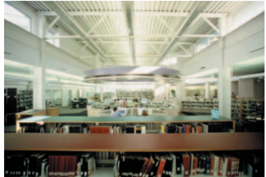
Photo sensors control the dimmable electric lighting to supplement the available daylight and maintain constant illuminance levels within the Harmony Library in Fort Collins, Colorado.
