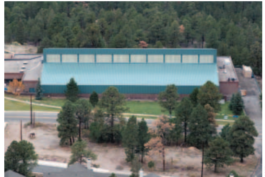
ENERGY STAR-compliant roof materials include metal and are applicable to both low-slope and steep-slope roof configurations.
