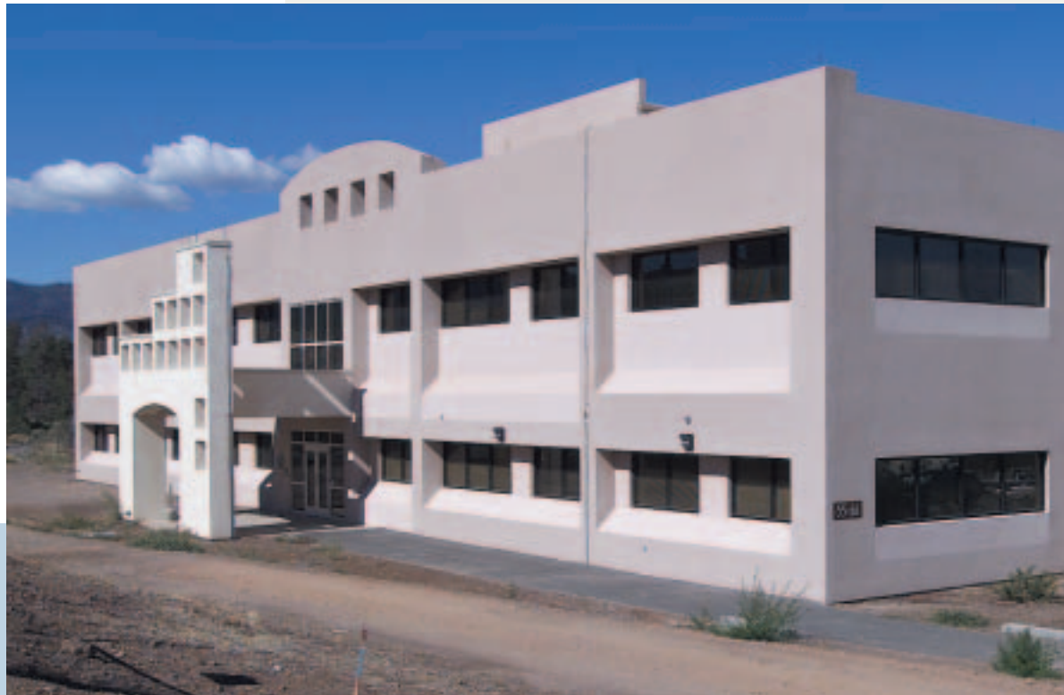
The architectural facade recesses surrounding the south-facing windows also serve as window overhangs to shade the windows and minimize direct solar gains. Placing the windows at the top of these recesses further enhances the effectiveness of these overhangs.
