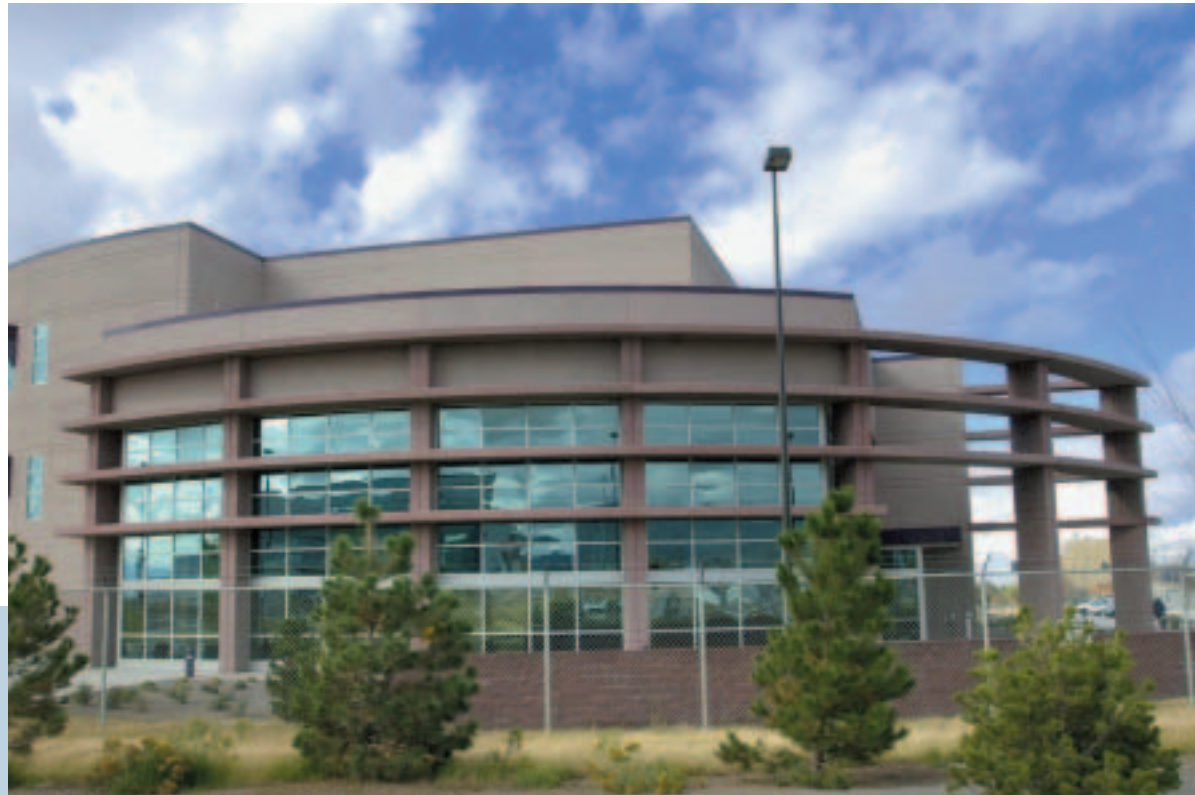
South facade, horizontal architectural elements to shade the atrium windows of the Process and Environmental Technology Laboratory, Sandia National Laboratories, Albuquerque, New Mexico. Exterior shading devices and light shelves can often be designed as prominent aesthetic architectural features.
