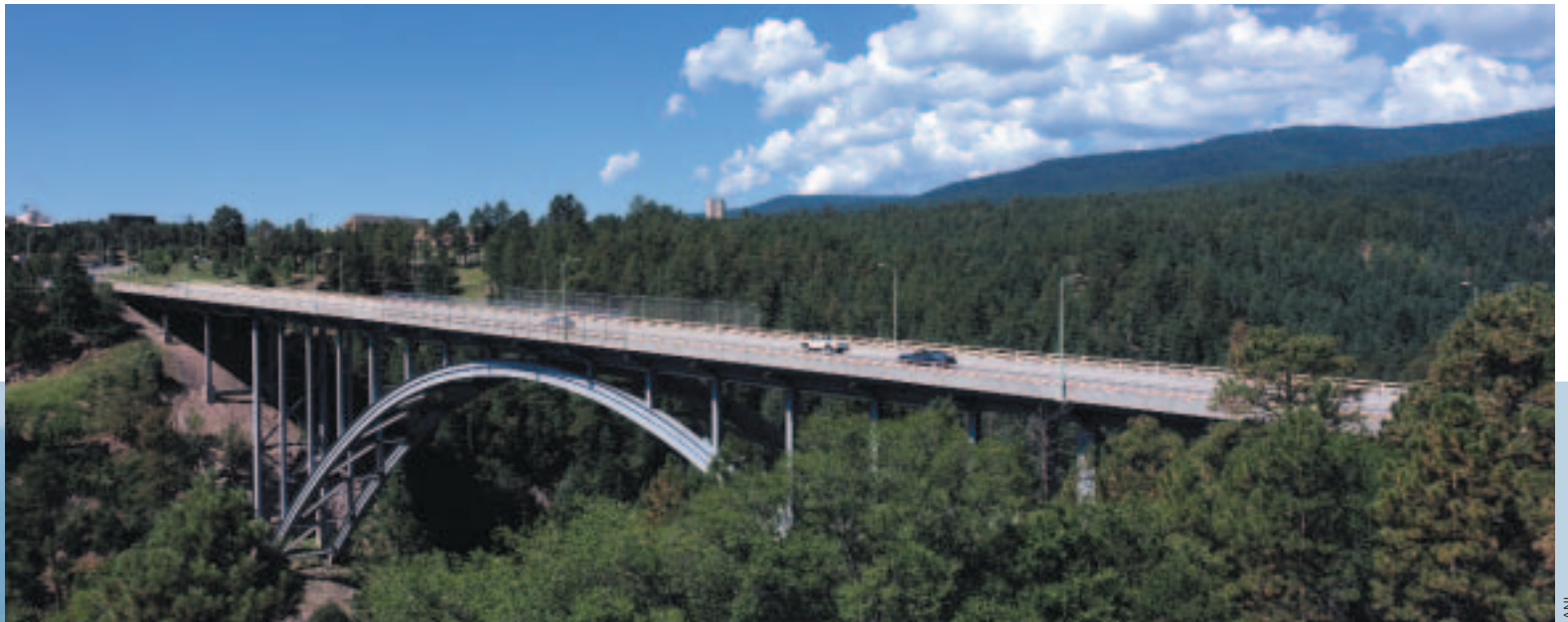
The Los Alamos Canyon Bridge opened the way for LANL growth onto the South Mesa.
