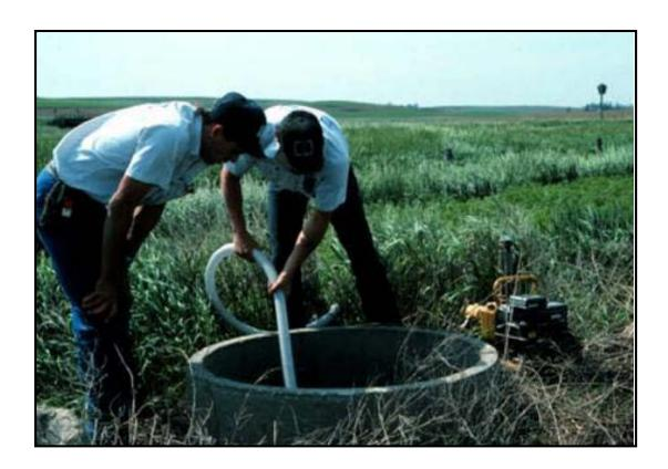
A vertical drain is a well, pipe, pit, or bore in porous underground strata into which drainage water can be discharged without contaminating groundwater resources.
