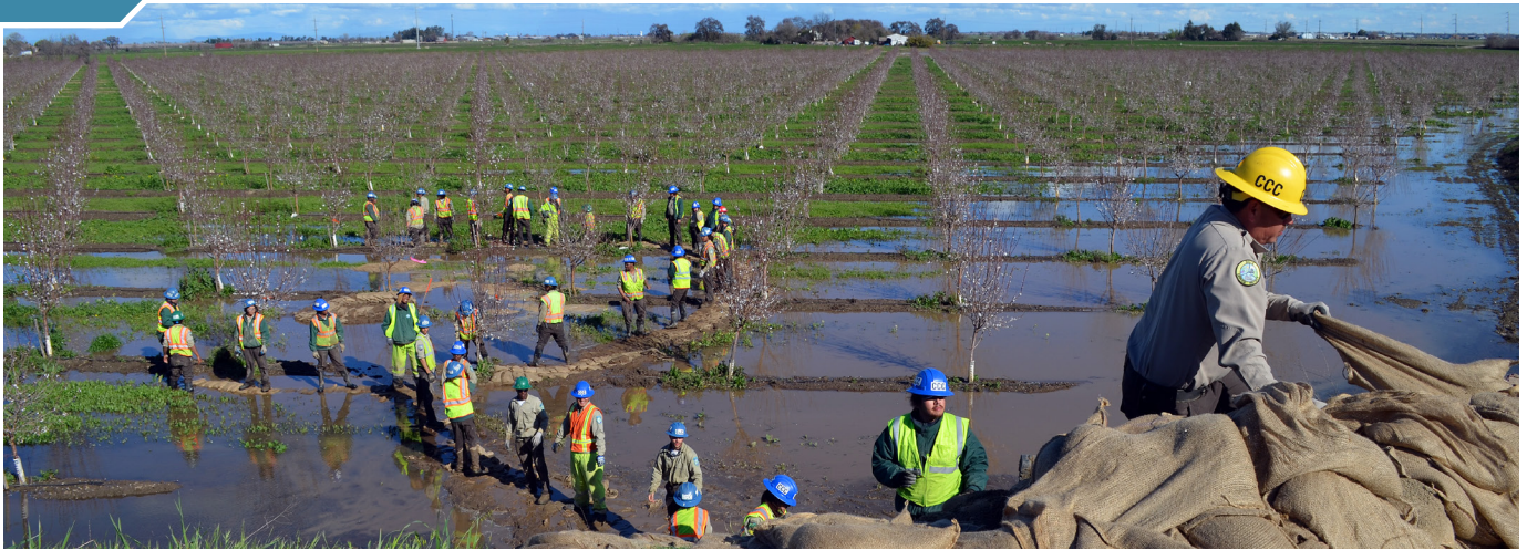
Levee repair along the San Joaquin River in California, February 2017
