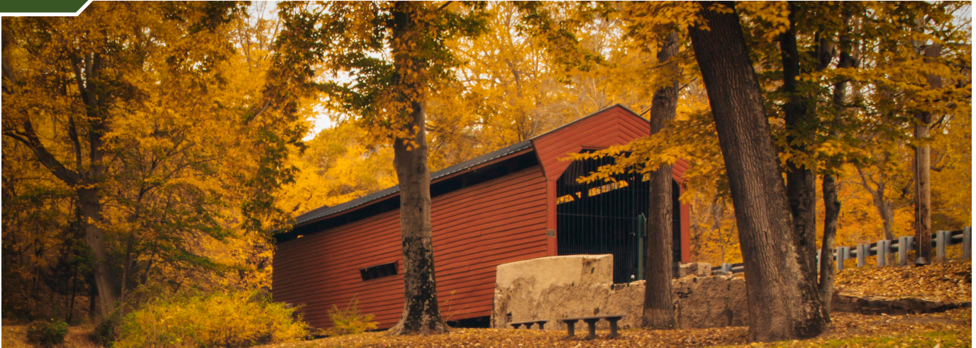
Bartram Bridge in Pennsylvania
