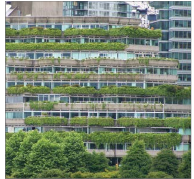
This residential building in Vancouver, Canada is covered in green decks to help mitigate the urban heat island effect. (Courtesy NNECAPA)
