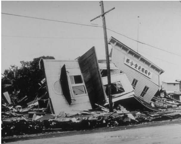
A building destroyed during the Hilo, Hawai'i, tsunami on April 1, 1946. Every house on the main street facing Hilo Bay was washed across the street and smashed against the buildings on the other side. (Image courtesy of NOAA and the U.S. Army Corps of Engineers)
