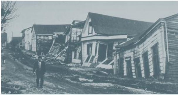
Considerable damage to quality, wood-frame houses in Valdivia, Chile occurred during the 1960 earthquake that shook southern Chile. Valdivia suffered catastrophic damage because of its proximity to the epicenter of the massive quake. (Image courtesy of NOAA, Pierre St. Armand, photographer)
