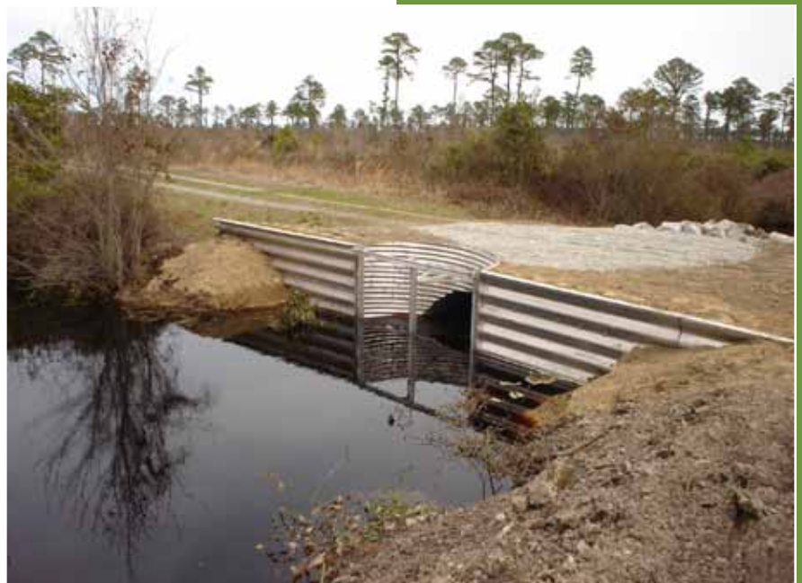
Water control structure at Great Dismal Swamp NWR.
