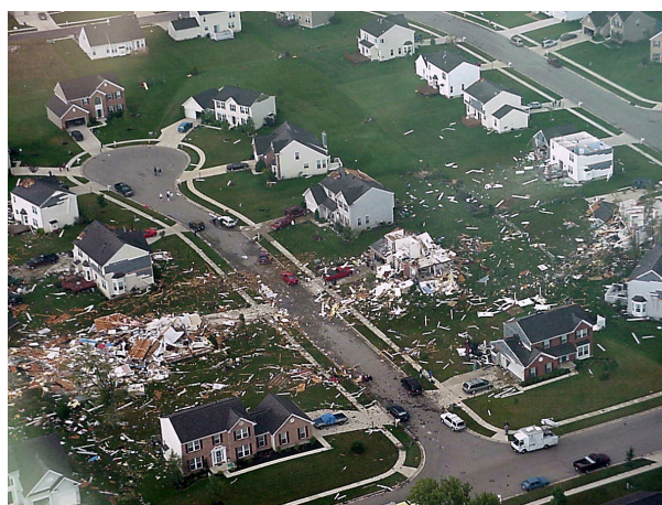
Figure 7a: Aerial view of damage from the Xenia, OH tornado, September 20, 2000.
