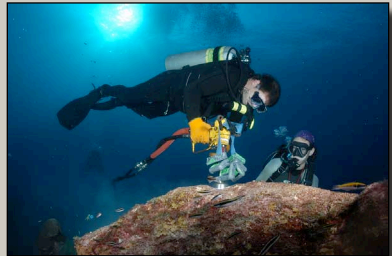
Installing mooring buoy anchors at the Flower Garden Banks NMS
