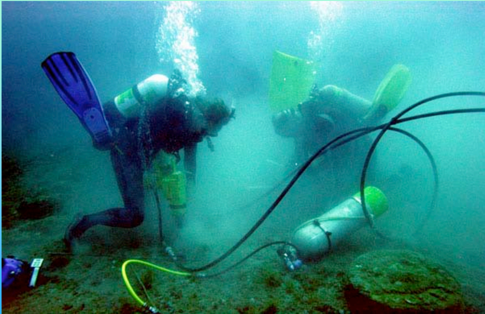
G. P. Schmahl and D. Haas installing new mooring buoy anchor
