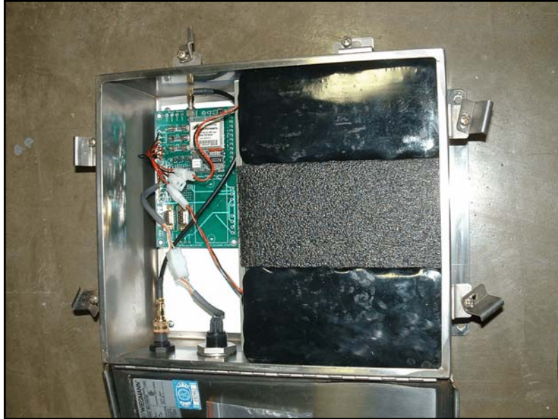
Figure 3. The ATON topside electronics box
