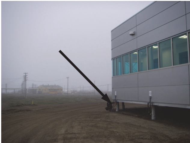
Figure 5a. Pilings on the Barrow Global Climate Change Research Facility were used as tidal bench marks.
