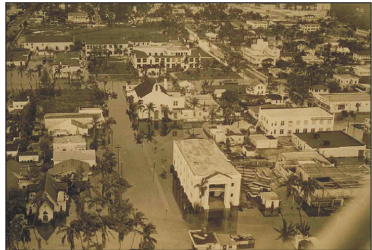
Figure 32. Photographs showing extensive flooding in (A) Hialeah and (B) Fort Lauderdale caused by major hurricanes that hit southeastern Florida in 1947 and 1948, respectively.
