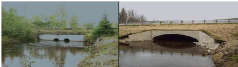
Figure 9a. Before: Prior to culvert structure.
