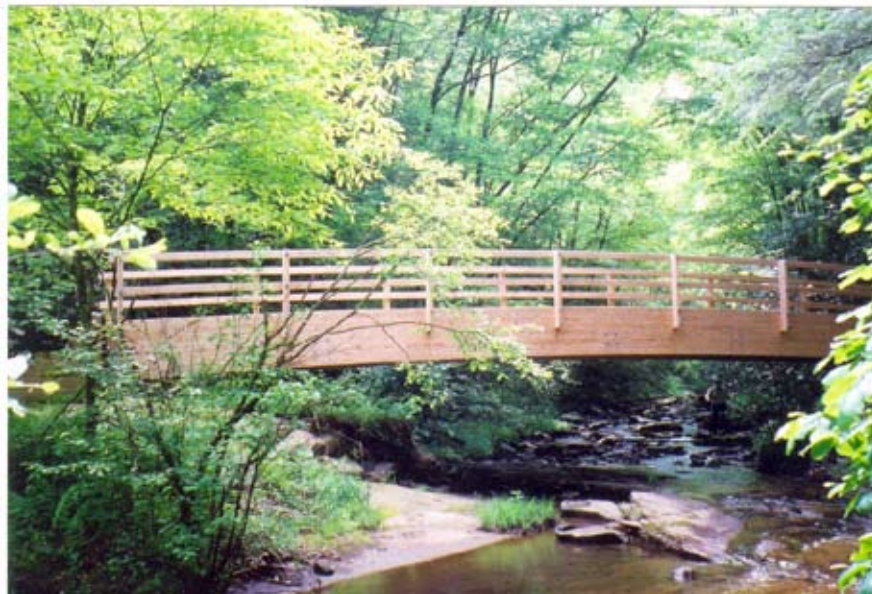
Figure 7. RTP funds helped pay for the construction of a bridge across Meadow Creek on the Monongahela National Forest.
