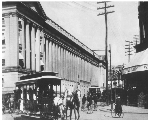
▲ The Treasury building in the late 1800s. The Treasury building colonnade from the southeast side shows the bustle of pedestrian traffic on 15th Street as they passed in front of the Treasury building.
