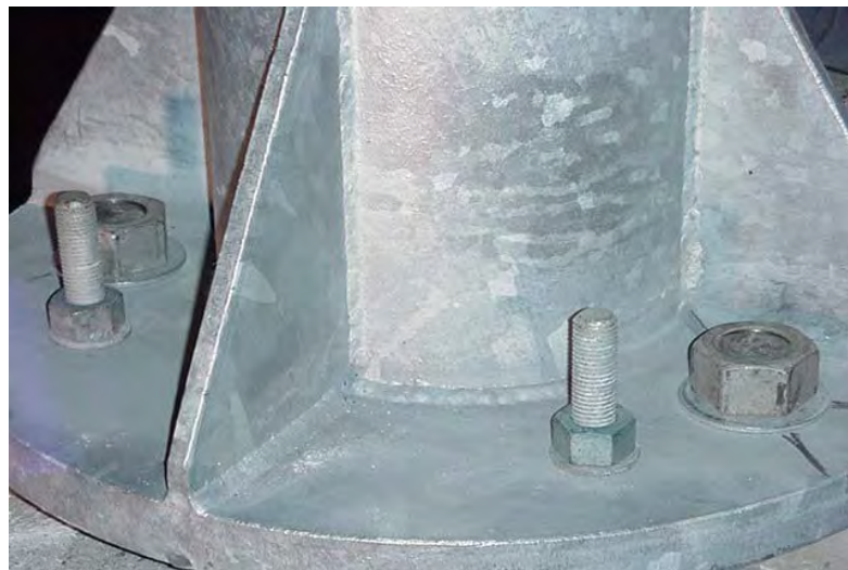
Figure 35. Base plate with Added Anchor Rods.
