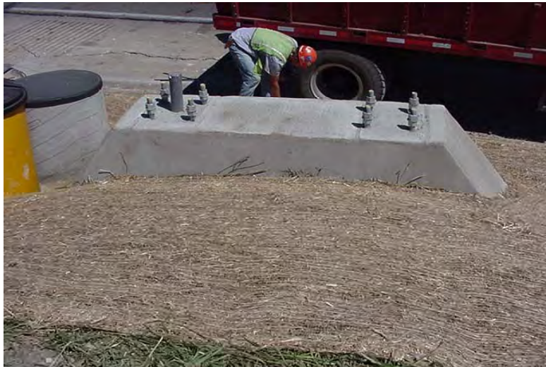
Figure 5. Foundation Ready for Structure Installation.
