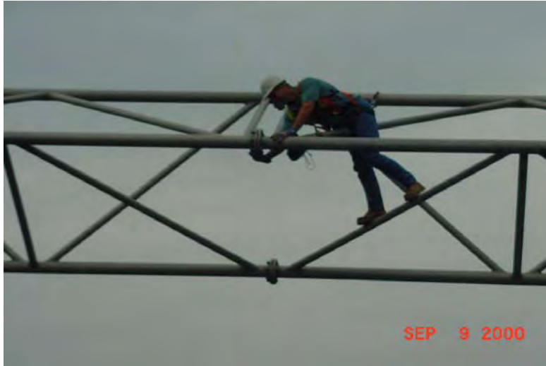
Figure 25. Hands on Inspection of Overhead Signs.
