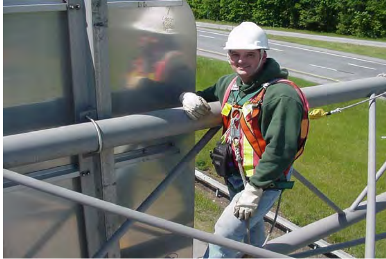
Figure 19. Inspector Uses Double Lanyard System.
