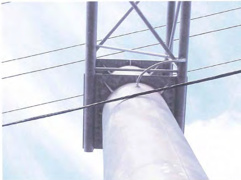
PHOTOGRAPH 4: COLUMN TO ARM CONNECTION
