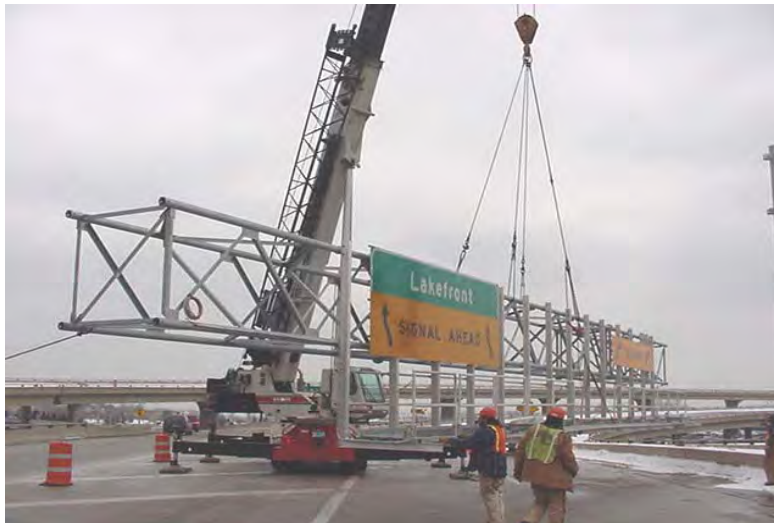
Figure 7. Assembled Truss Being Lifted Into Place.
