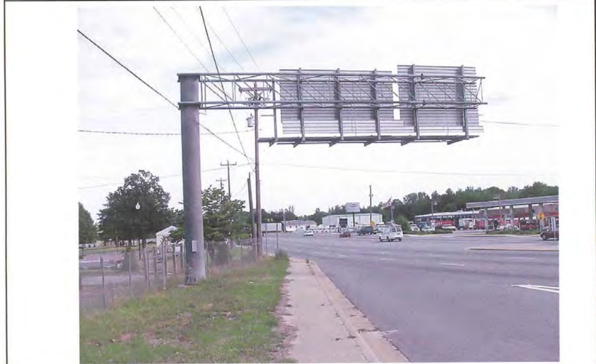
PHOTOGRAPH 2: BACK OF STRUCTURE
