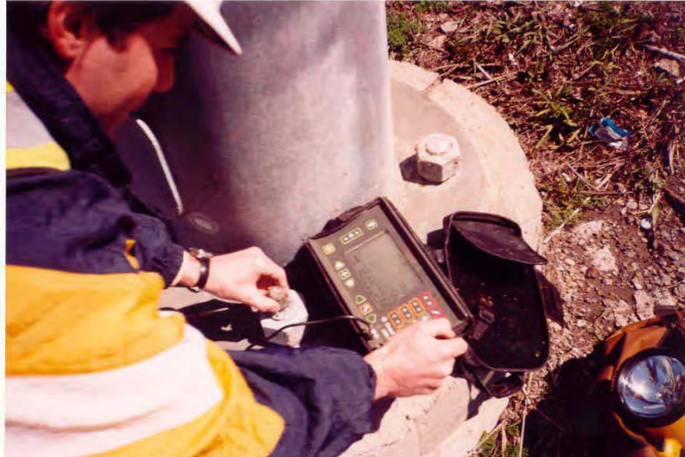
Figure 33. Ultrasonic Testing of Anchor Rods.
