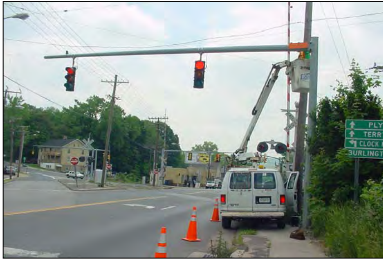
Figure 26. Inspection of a Mast Arm Structure.
