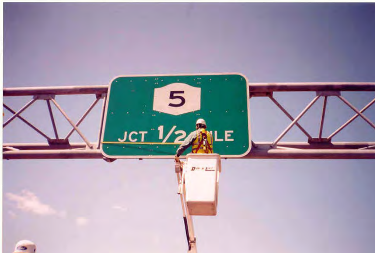
Figure 16. Inspector Measures Sign Panel During Inventory/Inspection Operation.
