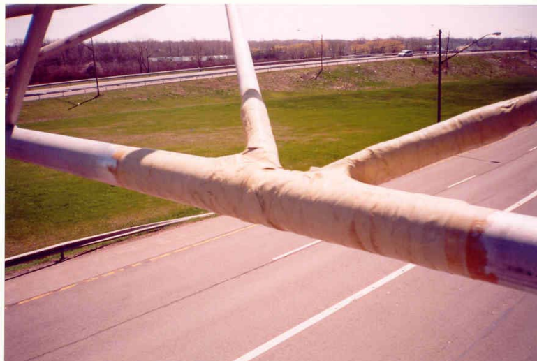
Figure 37. Repair of Truss Members Using FRP.
