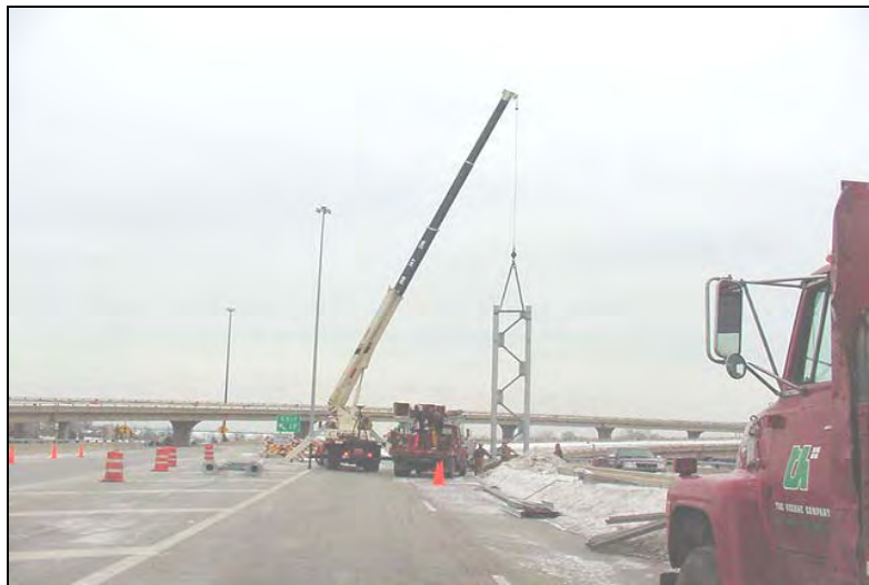
Figure 6. End Frame Being Set Onto Its Foundation.
