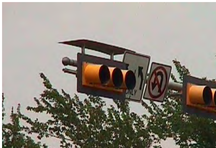
Figure 39. Texas Flat Panel Damper.
