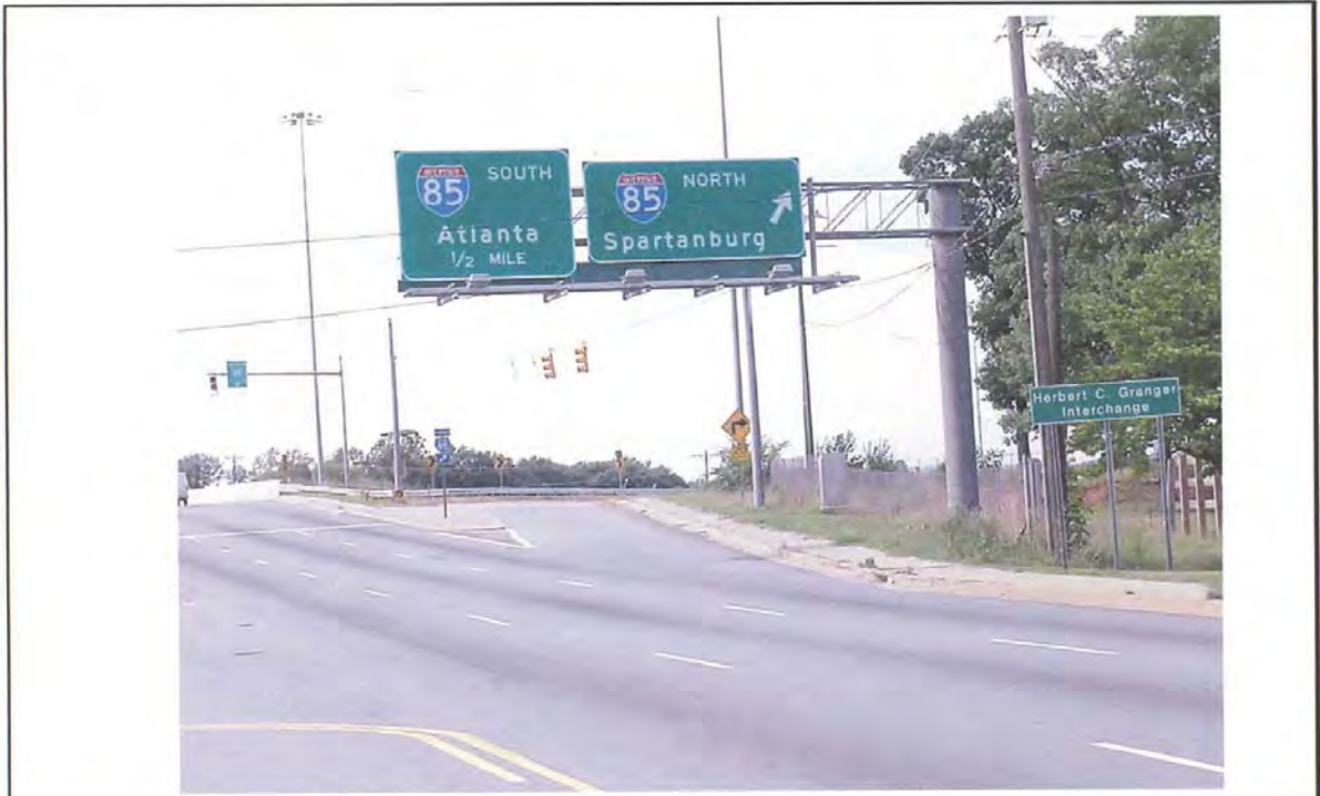
PHOTOGRAPH 1: FRONT OF STRUCTURE
