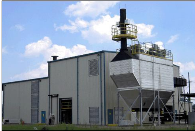
SRS's Biomass Steam Plant
