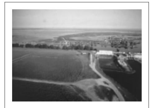
FIGURE 2 Water Control Structure
