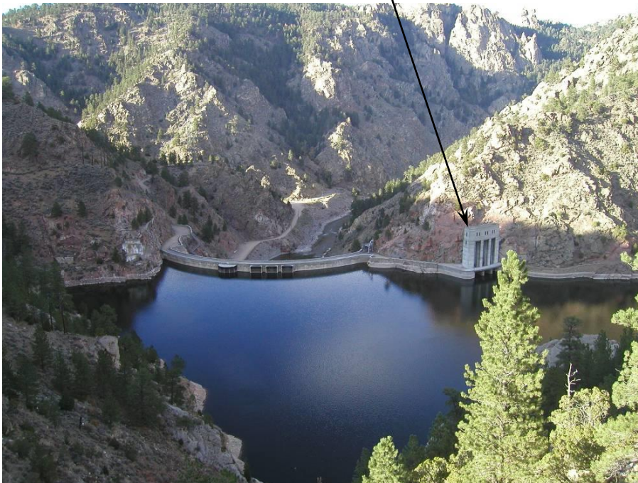
Tunnel inlet service spillway near right dam abutment, Seminole Dam, Wyoming
