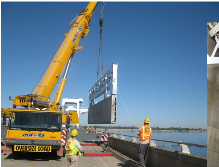
Folsom Dam, California: installation of metal stoplogs
