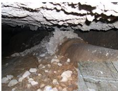
Big Sandy Dam, Wyoming - 1983 spillway chute stagnation pressure failure, exacerbated by excessive seepage and frost damage
