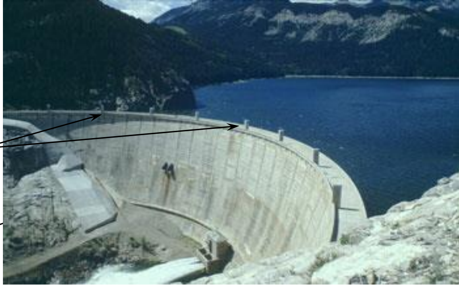
Overtopping protection for concrete dam (rockbolt and mass concrete armorment of right and left abutment and modified dam crest to serve as auxiliary spillway), Gibson Dam, Montana
