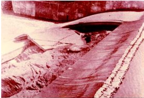
Big Sandy Dam, Wyoming - 1983 spillway chute stagnation pressure failure, exacerbated by excessive seepage and frost damage
