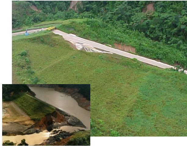
1999 Dam Failure due to Flood-induced Chute Wall Overtopping – El Guapo Dam, Venezuela (courtesy of Ing. Alejandro Hitcher).
