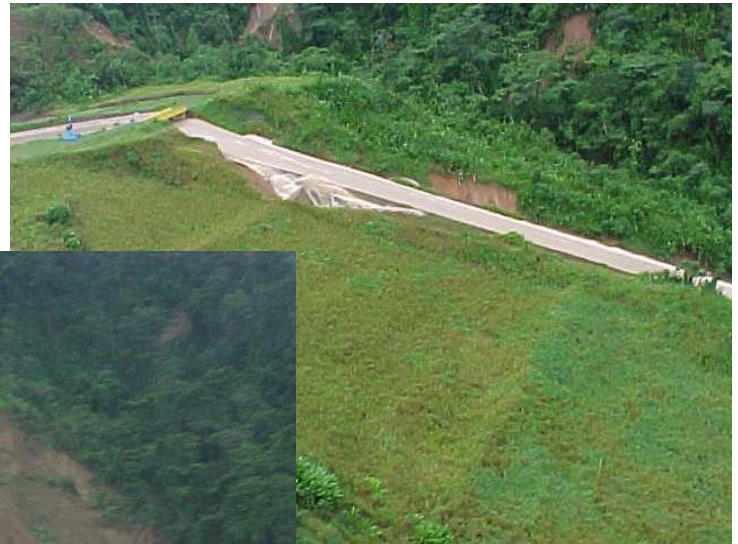
1999 spillway chute wall overtopping, leading to dam failure – El Guapo Dam, Venezuela (courtesy of Ing. Alejandro Hitcher).
