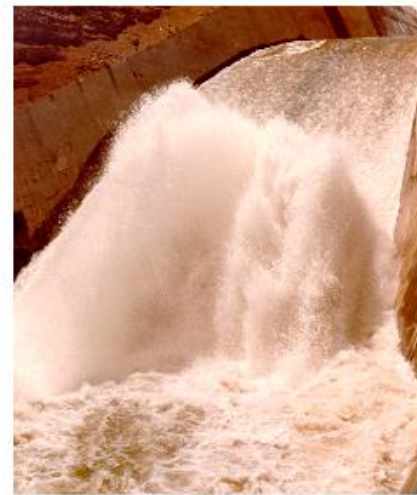
Big Sandy Dam, Wyoming - 1983 spillway chute stagnation pressure failure, exacerbated by excessive seepage and frost damage
