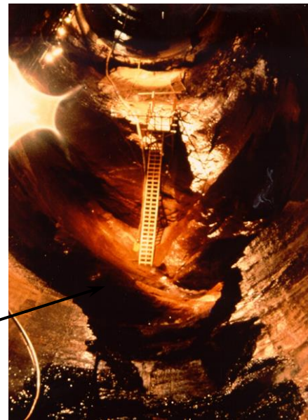
Figure 3.6.4.1.1-2. 1983 Spillway operations resulted in significant cavitation damage – Glen Canyon Dam, Arizona.
