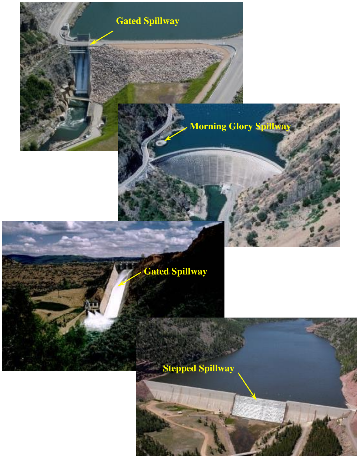
Figure 3.2.1.1-1. Service spillways, from top to bottom: Pineview Dam, Utah; Monticello Dam, California; Echo Dam, Utah; and Upper Stillwater Dam, Utah.
