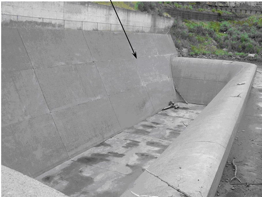
Side-channel service spillway, Paonia Dam, Colorado
