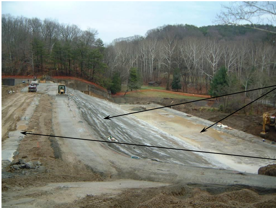
Overtopping protection for embankment dam (RCC armorment of dam and abutment), Vesuvius Dam (U.S. Forest Service), Ohio
