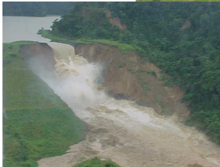
1999 spillway chute wall overtopping, leading to dam failure – El Guapo Dam, Venezuela (courtesy of Ing. Alejandro Hitcher).
