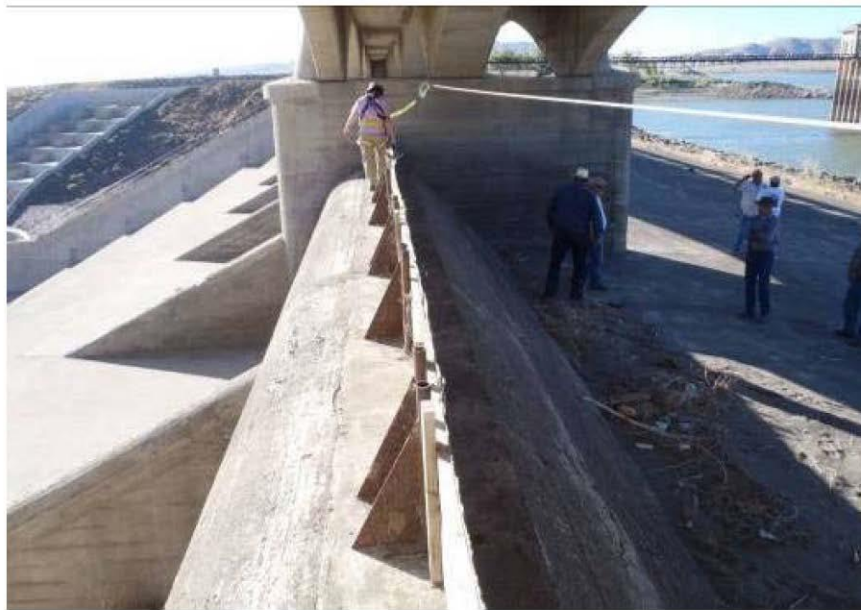
Figure 3.9.1.4-2. Flashboards – Lahontan Dam spillways.
