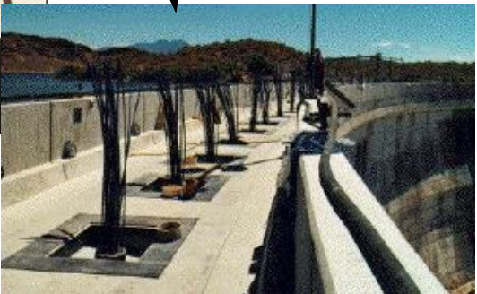
Stewart Mountain Dam Modifications, AZ – 1992 Stabilizing dam and modified existing river outlet works.
