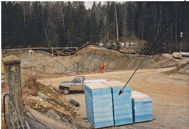
McDonald Dam (BIA), MT – 1995 New service spillway – Note ridge polystyrene insulating materials (stockpiled in upper photograph; installed on either side of waterstopped control joint, below reinforcement and above underdrains in right photographs).
