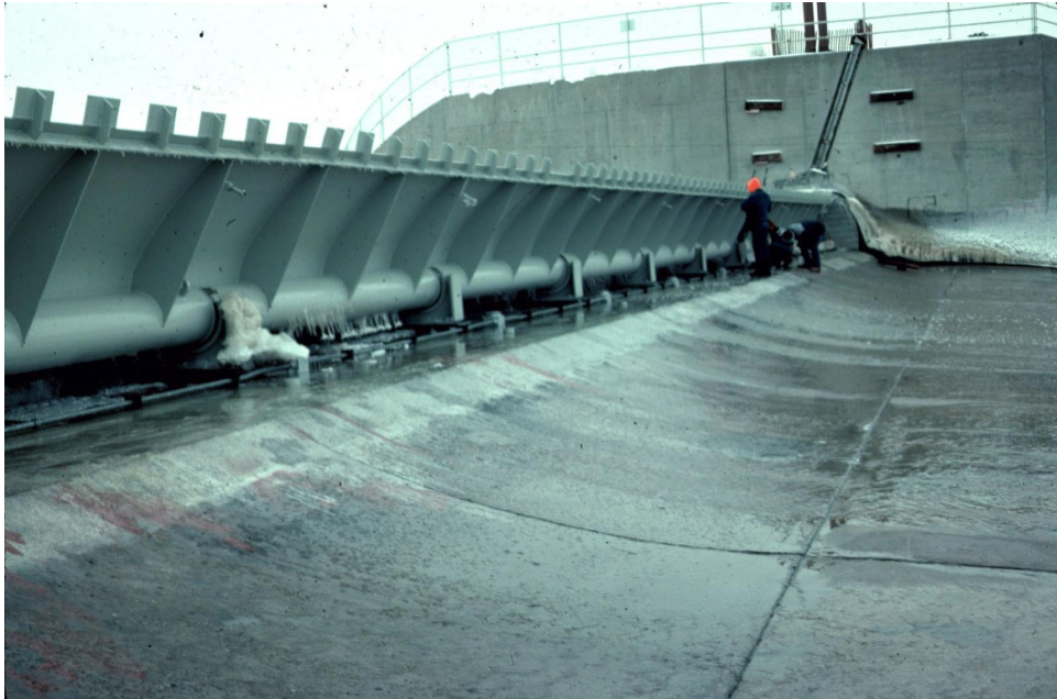
Figure 3.9.1.1-4. Crest gate – bascule type.
