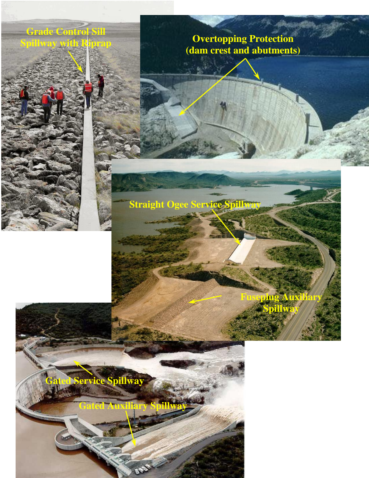
Figure 3.2.1.2-1. Auxiliary spillways, from top to bottom: Heart Butte Dam, North Dakota; Gibson Dam, Montana; New Waddell Dam, Arizona; and Stewart Mountain Dam, Arizona.
