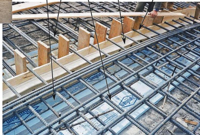
McDonald Dam (BIA), MT – 1995 New service spillway – Note ridge polystyrene insulating materials (stockpiled in upper photograph; installed on either side of waterstopped control joint, below reinforcement and above underdrains in right photographs).
