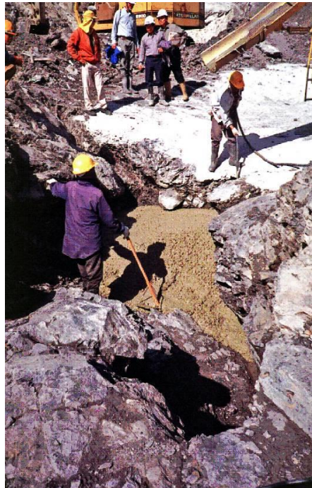
Treating foundation with dental concrete
