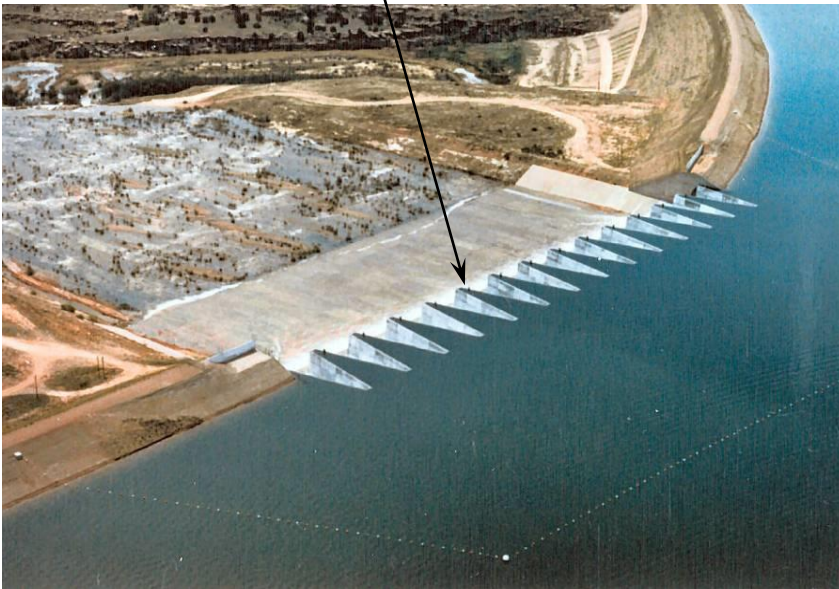
Labyrinth weir service spillway (New Mexico Interstate Stream Commission), Ute Dam, New Mexico
