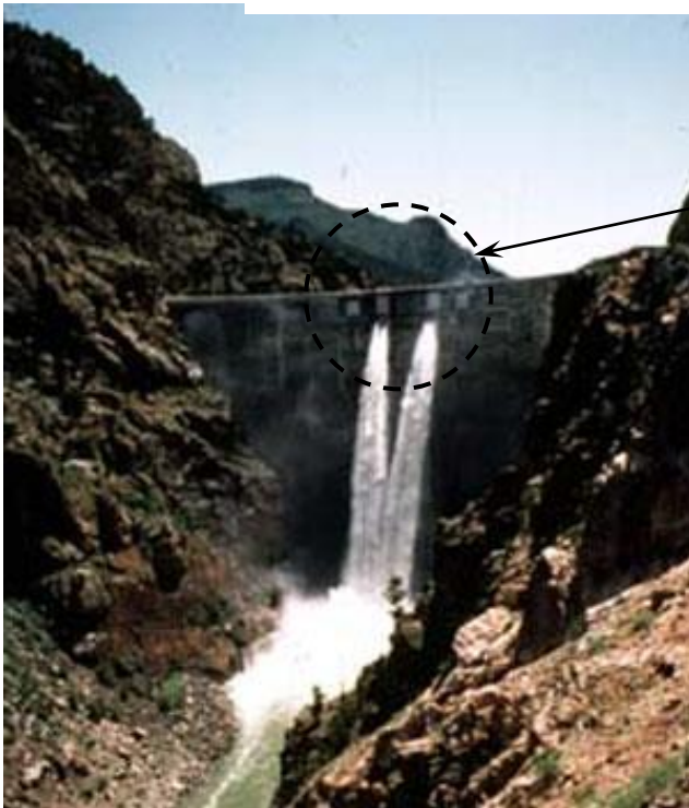
Orifice service spillway integral with concrete dam, Morrow Point Dam, Colorado
