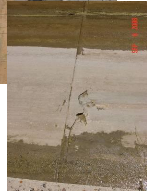
Spillway Chute Damage due to Thermo-expansion/contraction—Deer Creek Dam, Utah
