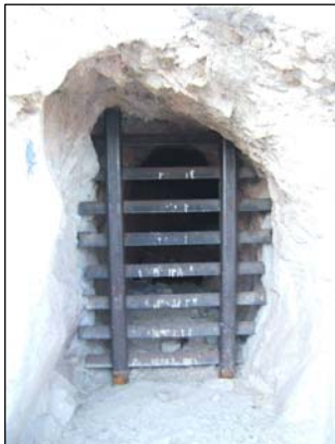
Figure 1. Example of a gated mine at the Salt Creek Hills Mine near Baker, CA
