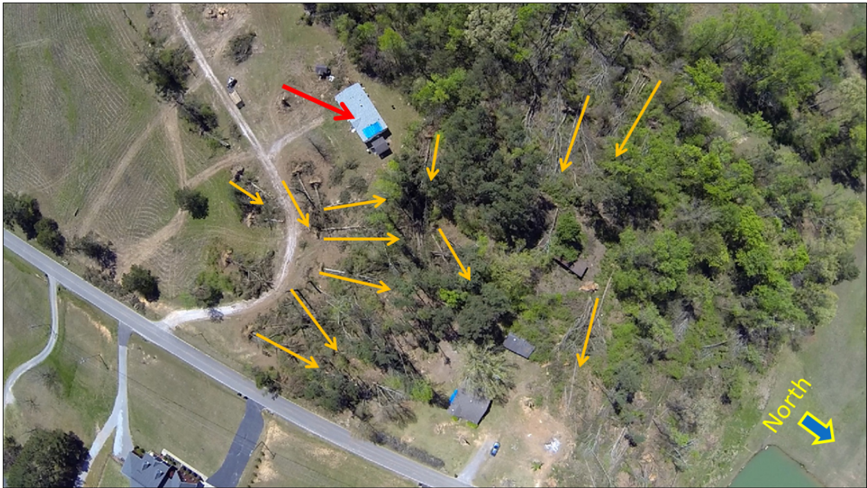
Figure 12: Damage near the middle of the Pricville tornado track on 5 April 2016 from Flight 2. Orange arrows indicate direction trees fell; red arrow indicates roof damage. North arrow indicated in bottom right.
