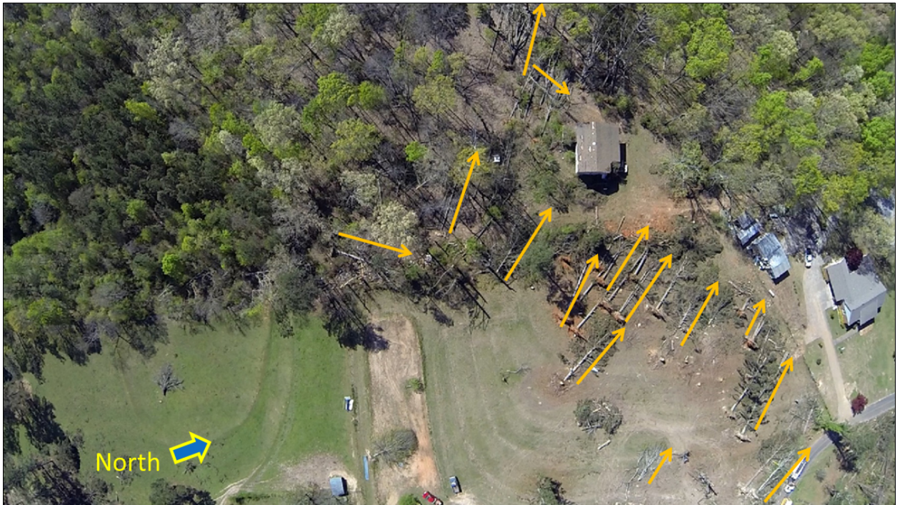
Figure 14: Damage near the middle of the Priceville tornado track on 5 April 2016 from Flight 4. Orange arrows indicate direction trees fell. North arrow indicated in bottom right.
