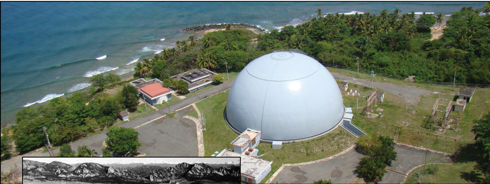
The decommissioned BONUS reactor facility is located on the westernmost coastal point of Puerto Rico in the municipality of Rincón.
