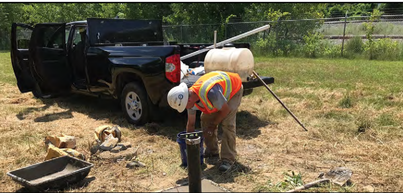
A worker repairs a damaged monitoring well.
