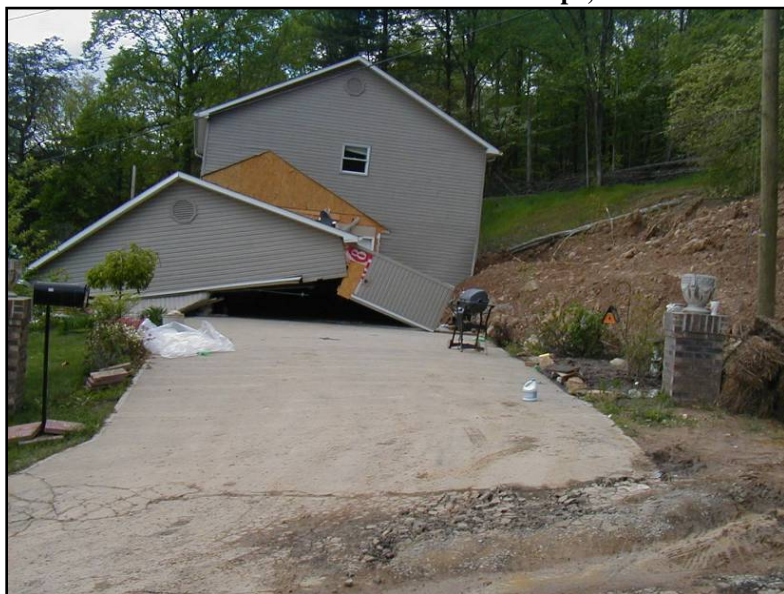
Figure 3.4-5 Destruction of a Residential Structure by a Landslide Caused by Human Activities (Excavation) into a Slope, Eastern Kentucky.
