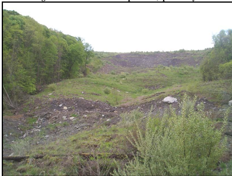
Figure 3.4-6 Failed Excess Spoil Fill (Specifically a Durable Rock Fill) in Eastern Kentucky
