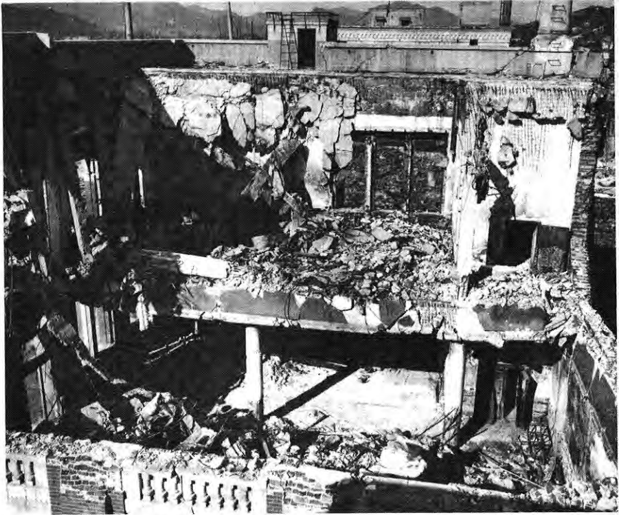
Figure 5.23. Reinforced-concrete building showing collapsed roof and floor slabs (0.10 mile from ground zero at Nagasaki).
