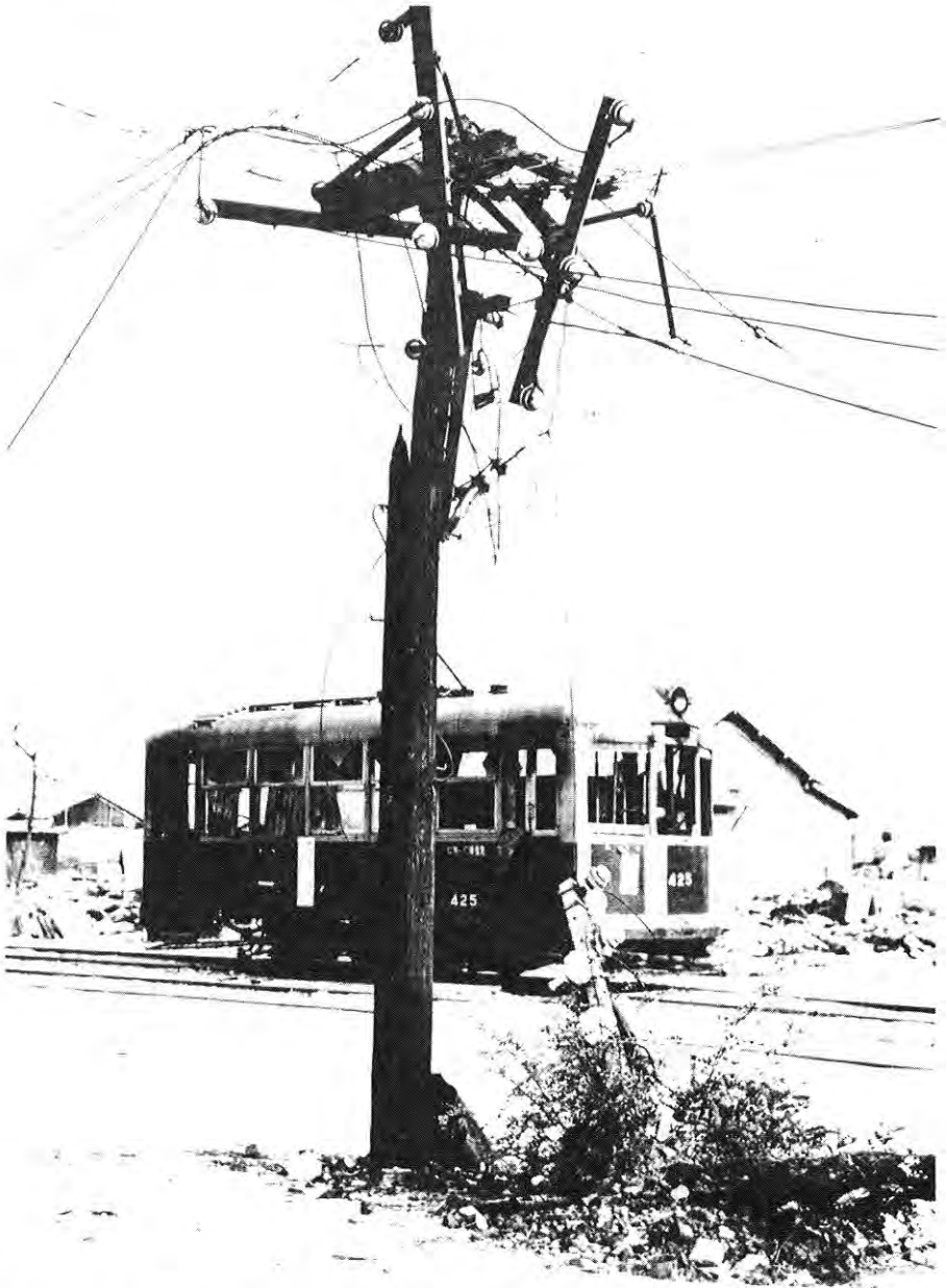
Figure 5.98. Damage to utility pole (0.80 mile from ground zero at Hiroshima).
