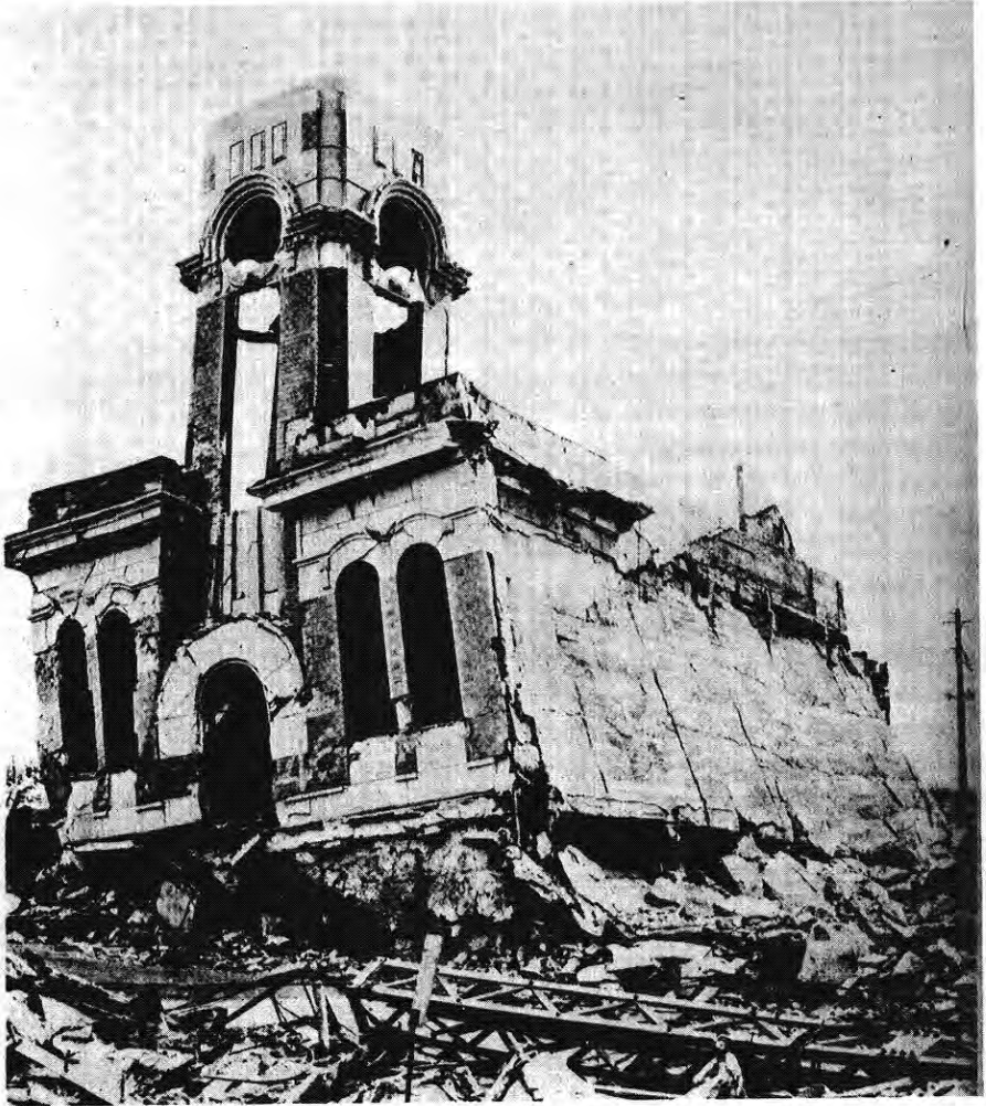
Figure 5.26. Two-story, steel-frame building with 7-inch reinforced-concrete wall panels (0.40 mile from ground zero at Hiroshima). The first story columns buckled away from ground zero dropping the second story to the ground.
