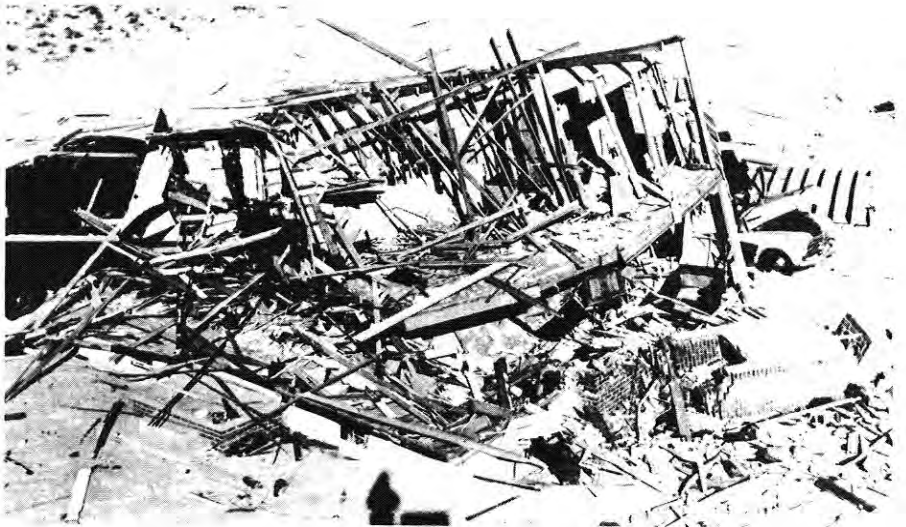
Figure 5.57. Wood-frame house after a nuclear explosion (5 psi peak overpressure).
