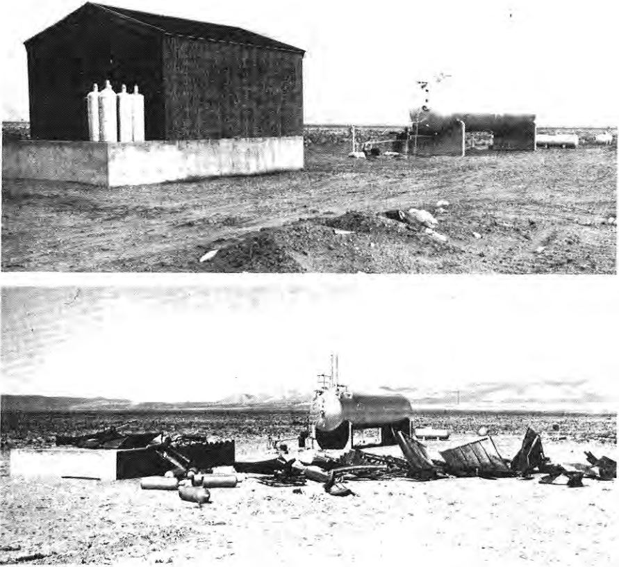
Figure 5.120. Upper photo: LP-gas bulk storage and filling plant before a nuclear explosion. Lower photo: The plant after the explosion (5 psi peak overpressure).
