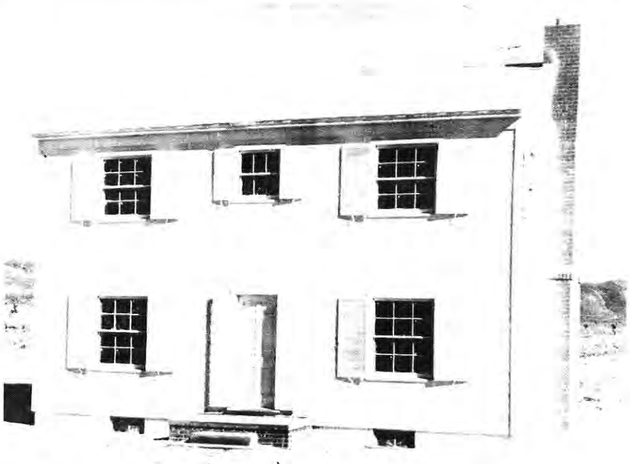
Figure 5.55. Wood-frame house before a nuclear explosion, Nevada Test Site.
