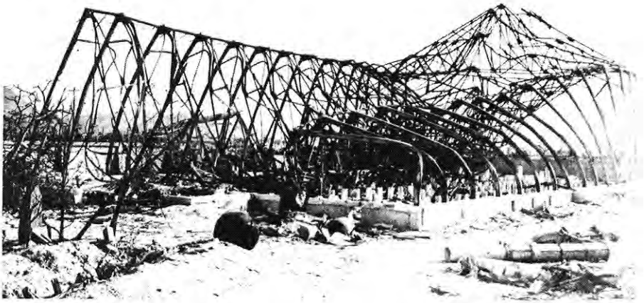
Figure 5.29. Single-story, light steel-frame building (0.80 mile from ground zero at Hiroshima); partially damaged by blast and further collapsed by subsequent fire.
