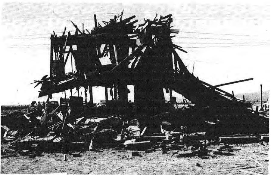
Figure 5.67. Unreinforced brick house after a nuclear explosion (5 psi peak overpressure).
