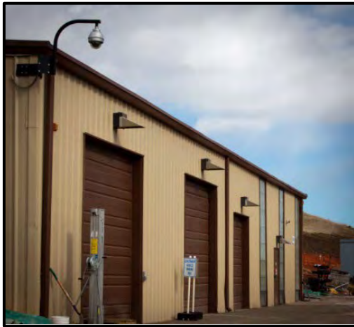
Facility Maintenance Building
