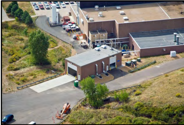
Renewable Fuel Heat Plant
