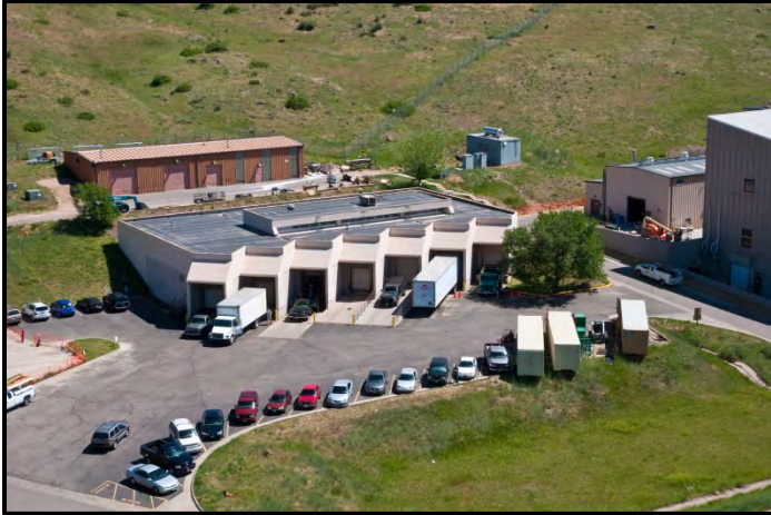
Shipping and Receiving Facility
