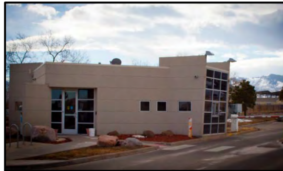
Site Entrance Building
