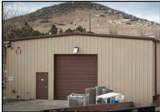
Bulk Storage Building
