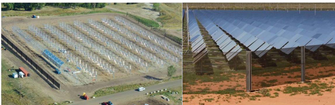
Figure 14. Wind and dust fences surrounding solar installations
