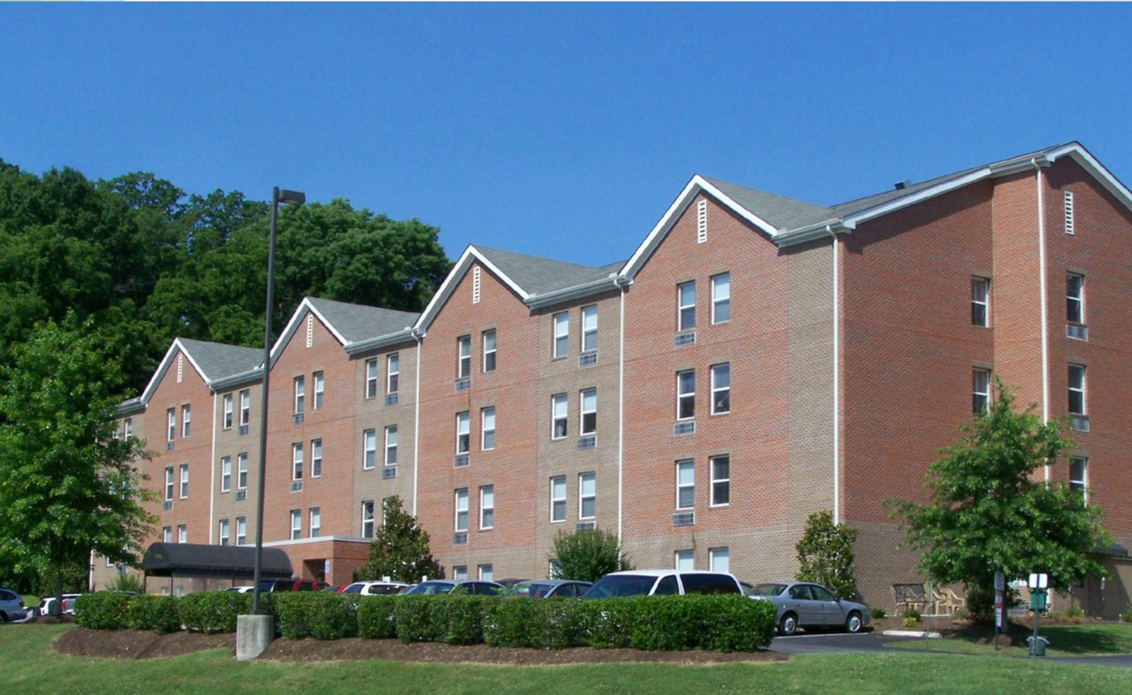
Heartland Christian Tower, Nashville, TN (Photo Credit: Staci Bergeron)
