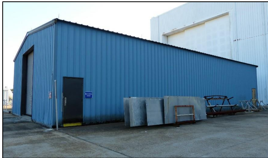
Figure 1-10. Mooring Storage Facility (Building 3203-A)
