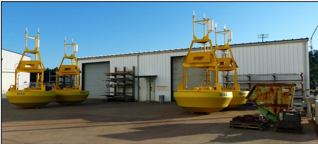
Figure 1-4. Welding Facility (Building 3208)
