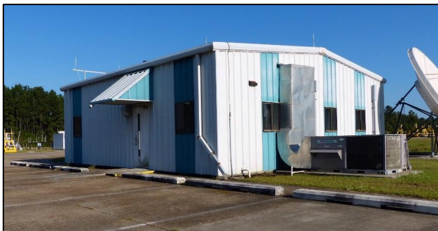
Figure 1-6. Ocean Sensor Calibration Laboratory (Building 3206)
