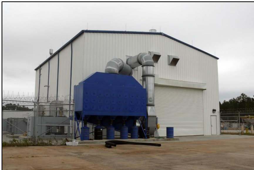
Figure 1-5. Paint and Sandblasting Facility (Building 3216)
