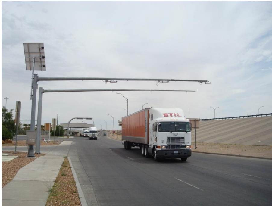
Figure 26. Photo. Truck leaving the State inspection facility on the US side of the border and passing under the RFID reader station.
