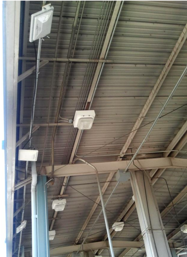
Figure 32. Photo. Completed installation of RFID equipment at CBP primary booth at BOTA.
