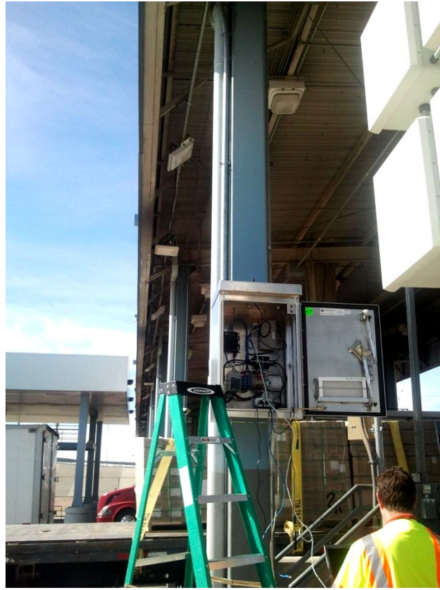
Figure 31. Photo. RFID equipment being installed at CBP primary booth at BOTA.
