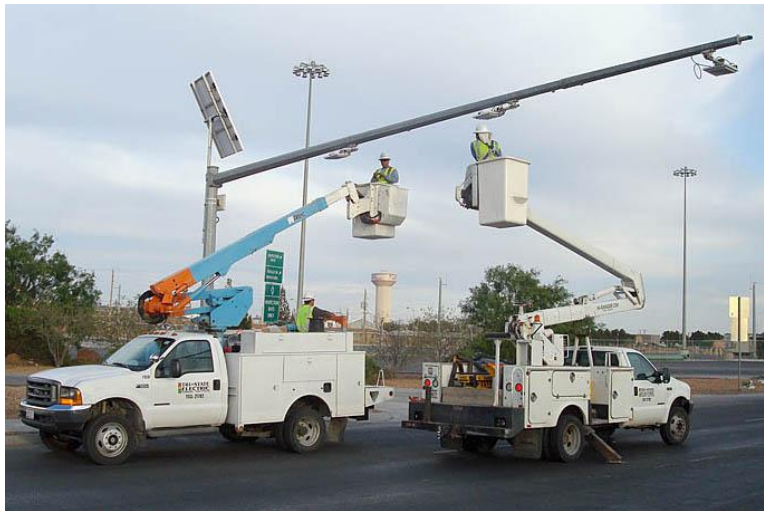
Figure 21. Photo. Contractors installing RFID antennae on a mast arm.
