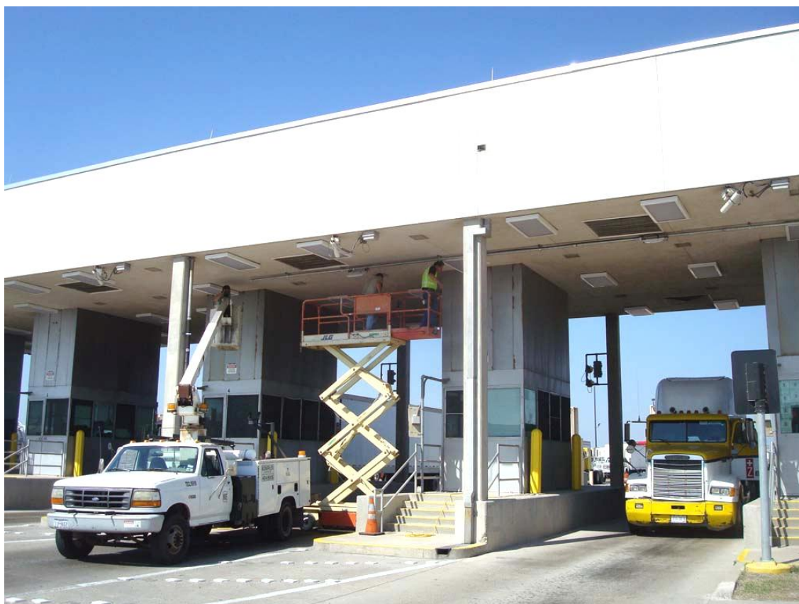
Figure 35. Photo. Contractors installing RFID equipment at CBP’s primary inspection facility at Pharr-Reynosa border crossing.
