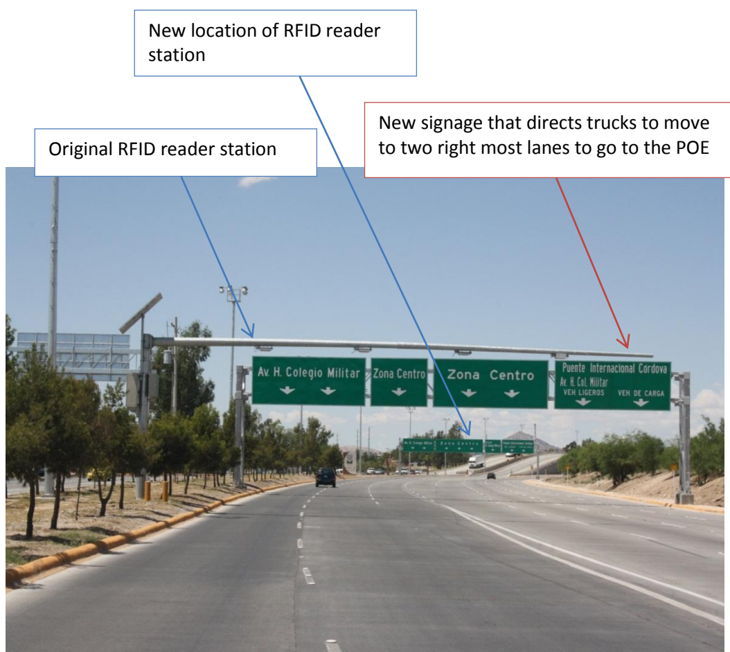
Figure 28. Photo. Original RFID reader station and new signage for relocation of original RFID equipment on the MX side of the BOTA.
