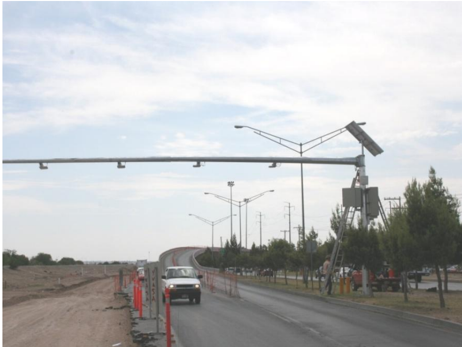
Figure 22. Photo. RFID antennae at the convergence of Boulevard Cuatro Siglos and MX45.
