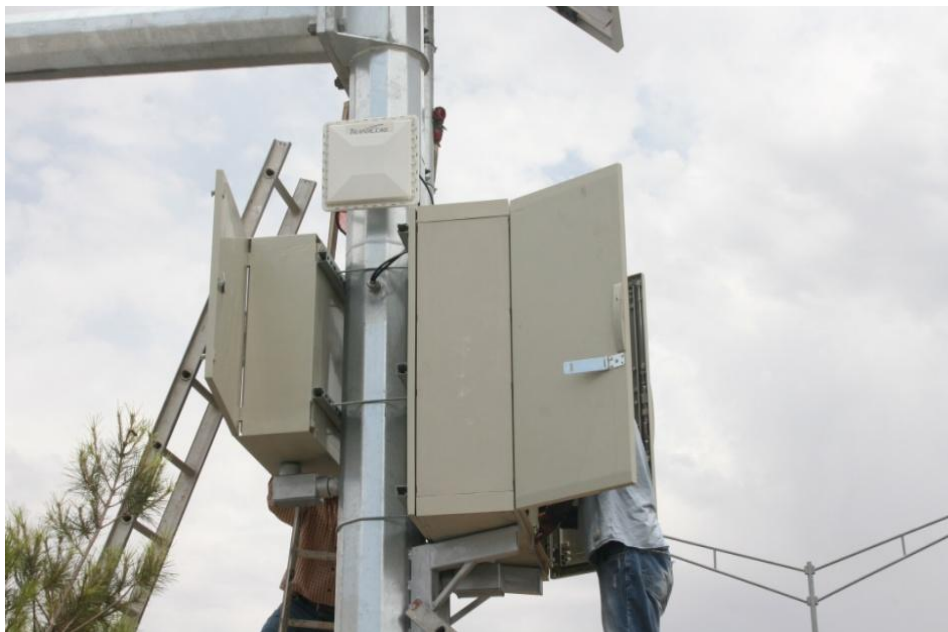
Figure 23. Photo. Contractors installing cabinets on a pole in Ciudad Juárez, Mexico.
