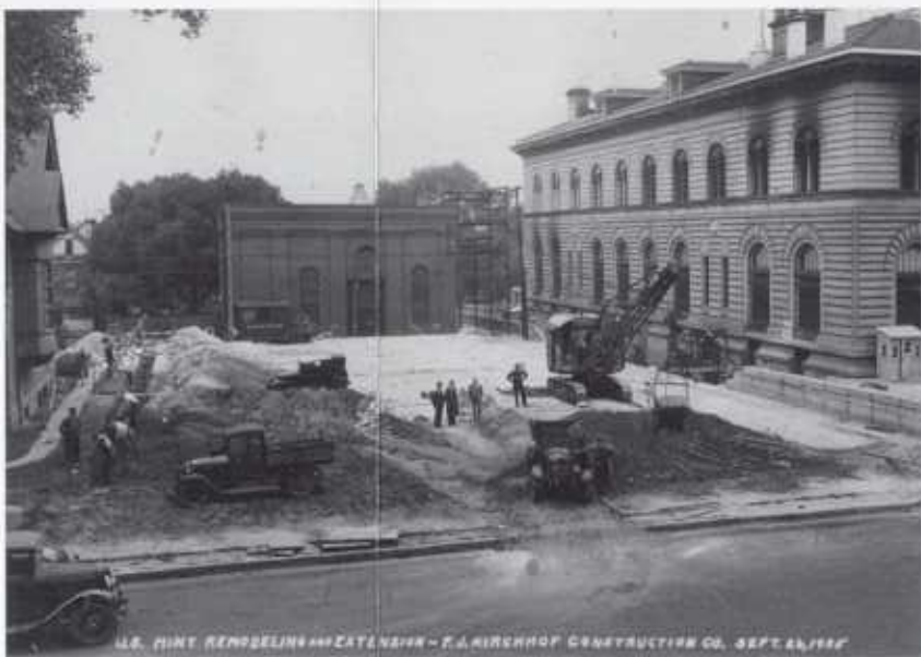
Construction at the Denver Mint, 1935. RG 104
