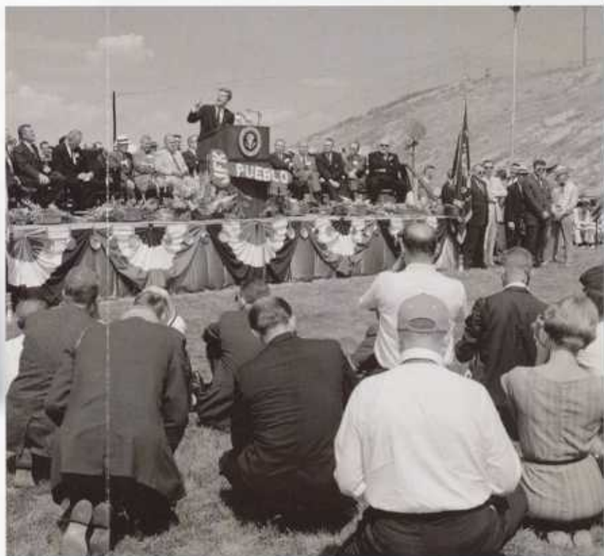
President John F. Kennedy at the dedication of the Fryingpan-Arkansas Project, Colorado, August 17, 1962. RG 115
