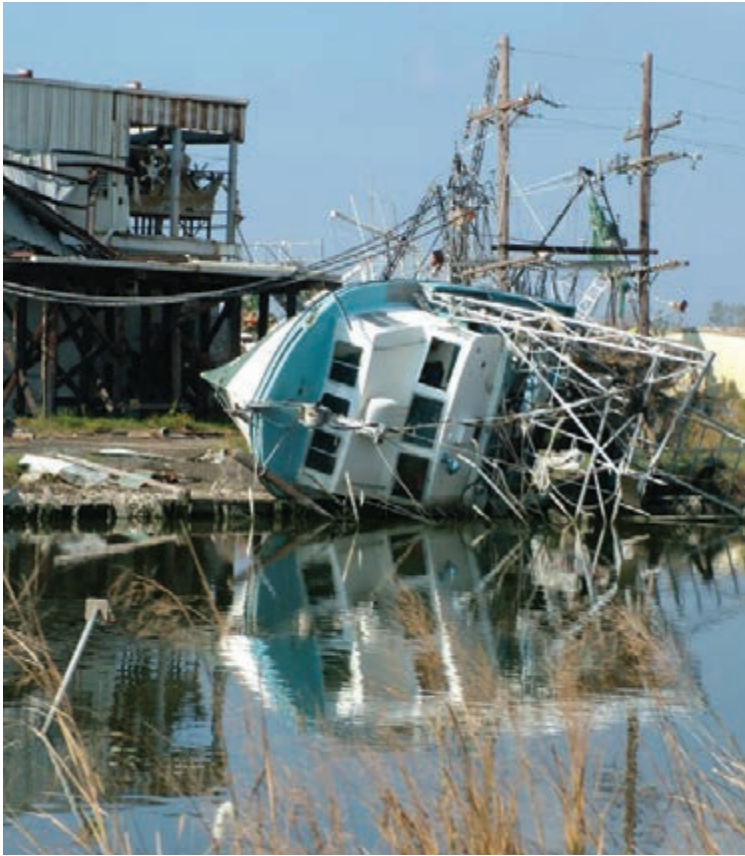
Figure 9.1 A fishing vessel lies on its side near a wholesale fishing dock in St. Bernard Parish, Louisiana, after Hurricane Katrina. Adjacent infrastructure also suffered massive damage. Photo by Paula Ouder. Courtesy of Louisiana Sea Grant College Program.
