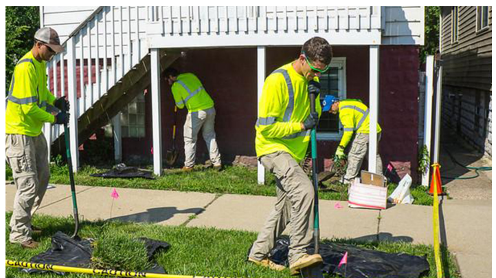
Soil cleanup on a residential property.
