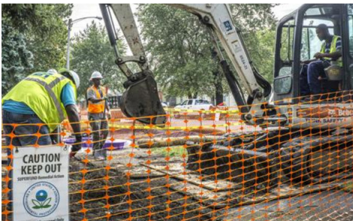
Soil cleanup of a Superfund site.
