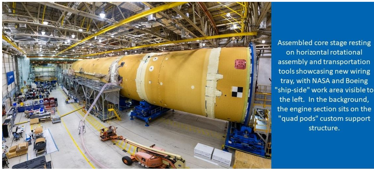
Figure 9: Core Stage Process Improvements at Michoud
