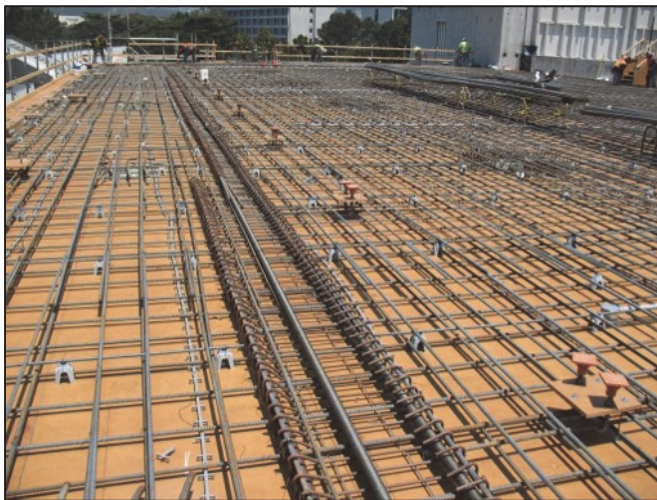
Figure 9-2. A long collector with confinement reinforcement.
