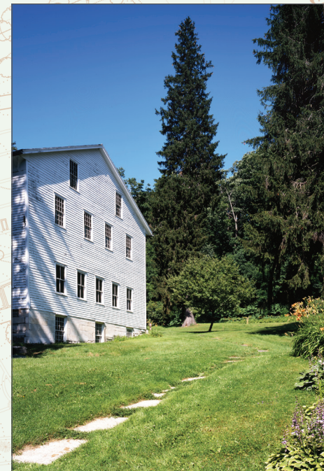
North Family, Mount Lebanon Shaker Village, New Lebanon, New York; view east from left to right of the Sister's Shop, stone walkway, and daylilies and hostas growing along the north side of the Second Dwelling House; James W. Rosenthal and Renee Bieretz, photographers, 2009.
